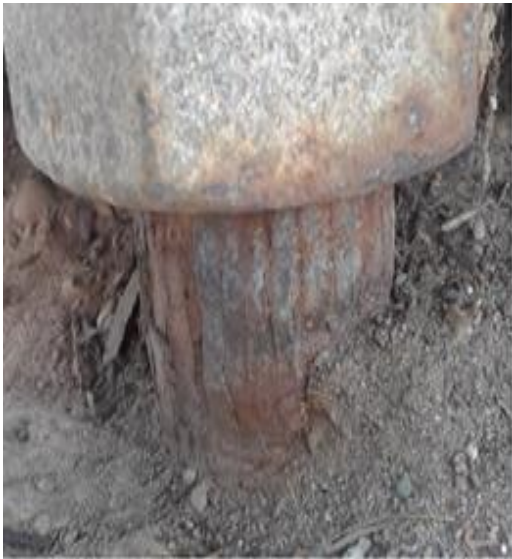
Figure 10-7: Anchor bolts and leveling nuts, anchor nut without fully engaged threads
