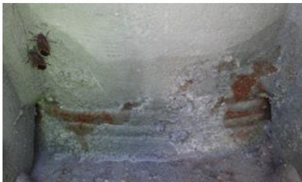
Figure 10-10: Corrosion in bonding clamp along bolt of base plate stiffener
