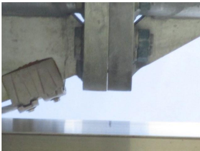
Figure 10-15: Horizontal structure connection, gap between arm connection flanges
