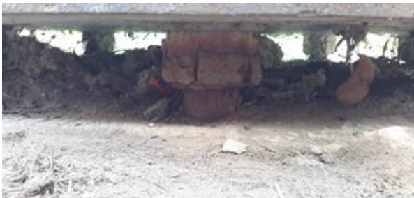
Figure 10-8: Leveling nut and anchor bolt corrosion with section loss
