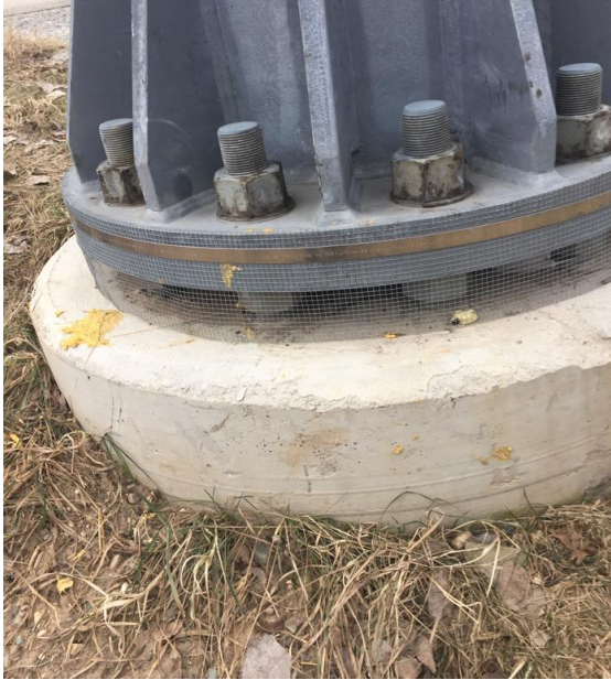
Figure 10-4: DMS support structure foundation, minor spalling
