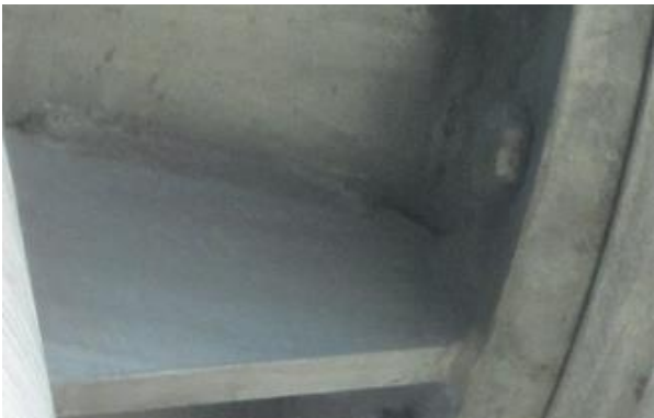
Figure 10-13: Vertical structure connection, loose bolt/lock washer not fully compressed
