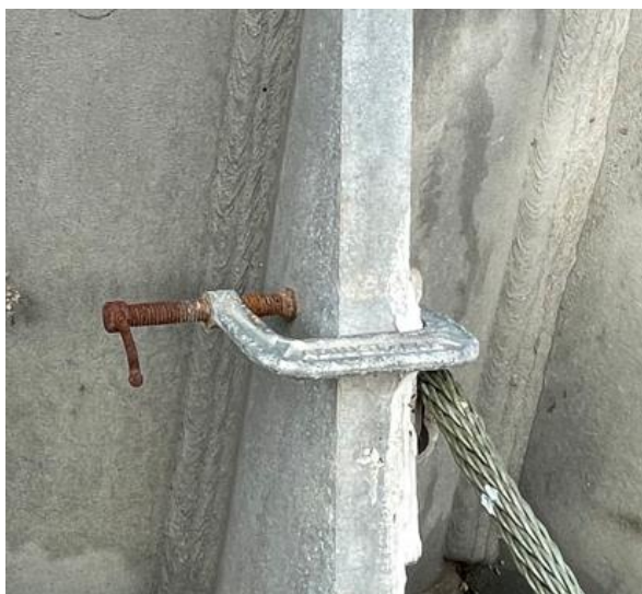
Figure 10-10: Corrosion in bonding clamp along bolt of base plate stiffener
