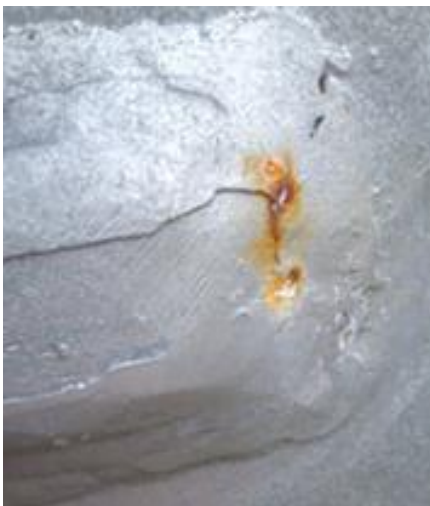
Figure 10-14: Vertical structure connection, rust bleeding through galvanizing at welded gusset plate arm to vertical structure upright
