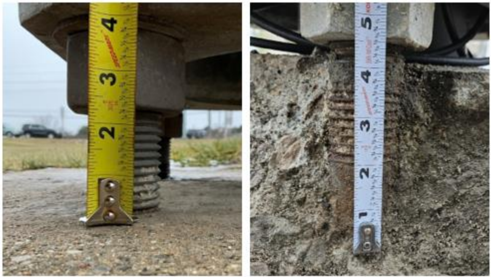
Figure 11-7: Standoff measurement for a sound foundation (left) and standoff measurement with foundation concrete deterioration (right)
