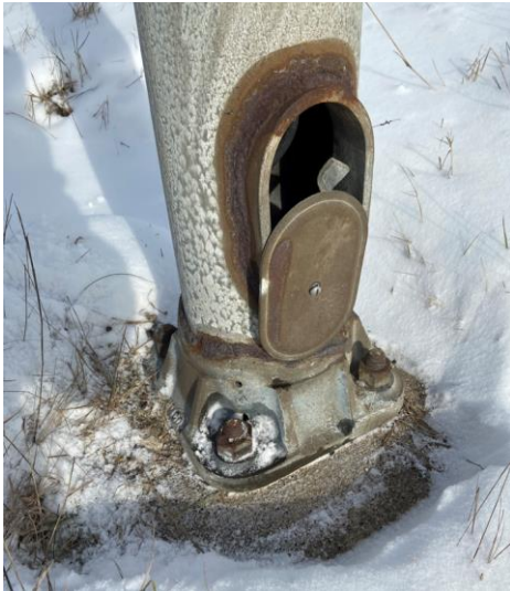
Figure 11-21: Non-frangible pole structure vertical support column (upright), visual identification of out of plumb pole (left), measurement of pole plumbness (right)
