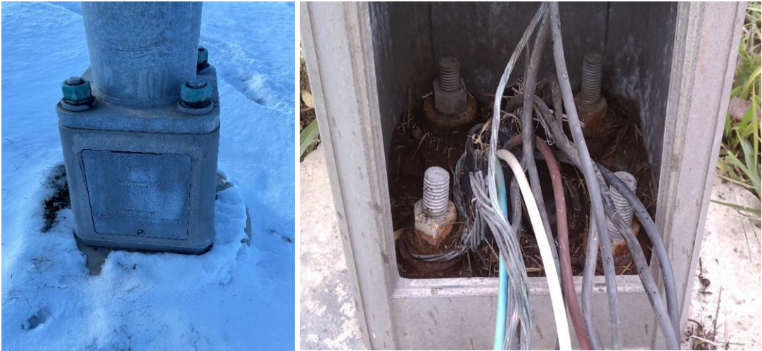
Figure 11-13: Frangible transformer base, panel door present (left), corrosion and debris in transformer base interior with missing panel door, and exposed wires (right)
