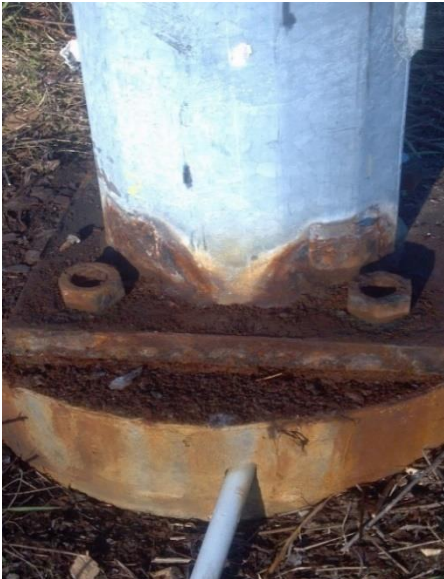
Figure 11-16: Non-frangible pole structure base plate, corrosion of base plate, anchor bolts, and nuts and inadequate bolt projection
