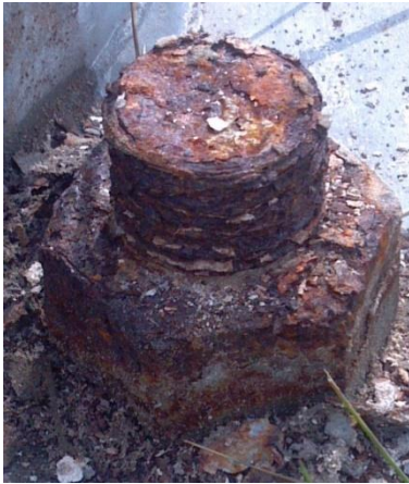
Figure 11-10: Anchor bolt and leveling nuts foundation, non-frangible base anchor bolt corrosion
