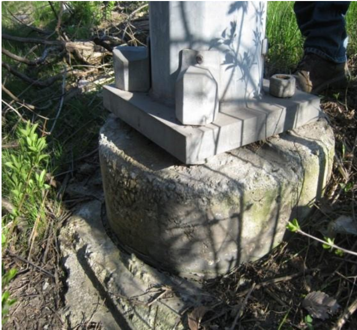
Figure 11-5: Non-frangible concrete foundation deterioration
