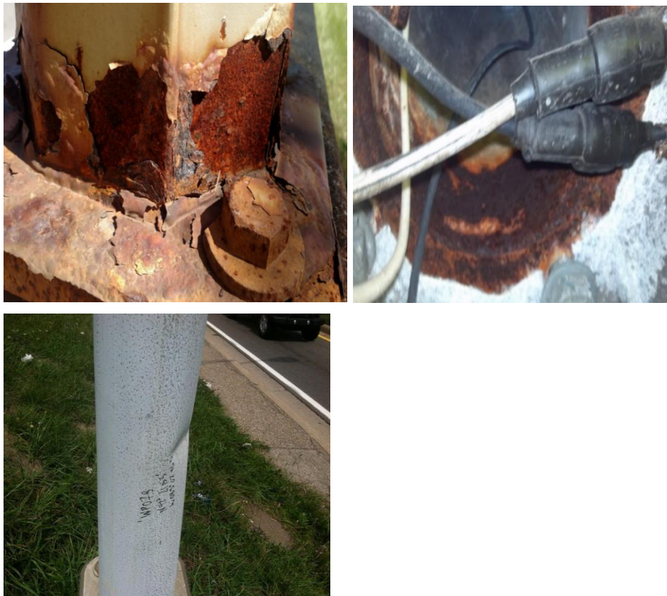
Figure 11-19: Non-frangible pole structure vertical support column (upright), dent
