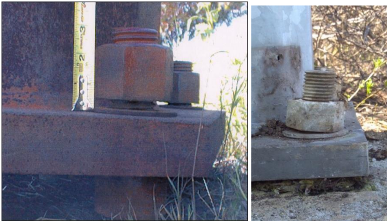
Figure 11-11: Anchor bolt and leveling nut foundation, gap between anchor nut and washer in corroding base unit (left), gap between anchor nut and washer with bolt out of plumb and debris between upright base and concrete foundation (right)
