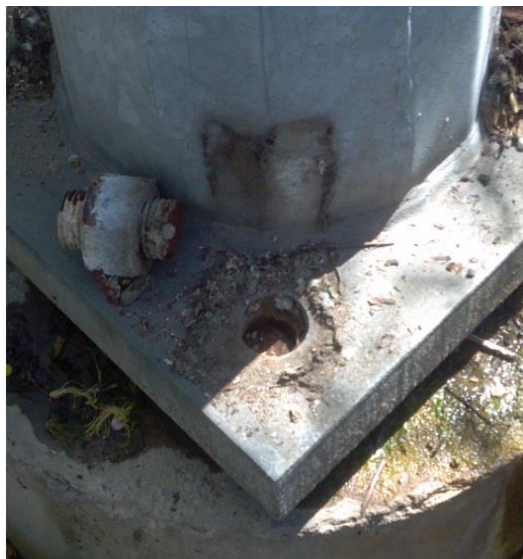
Figure 11-9: Frangible pole structure anchor bolts and leveling nuts foundation, loose anchor bolt (left), anchor nut without fully engaged thread (right)
