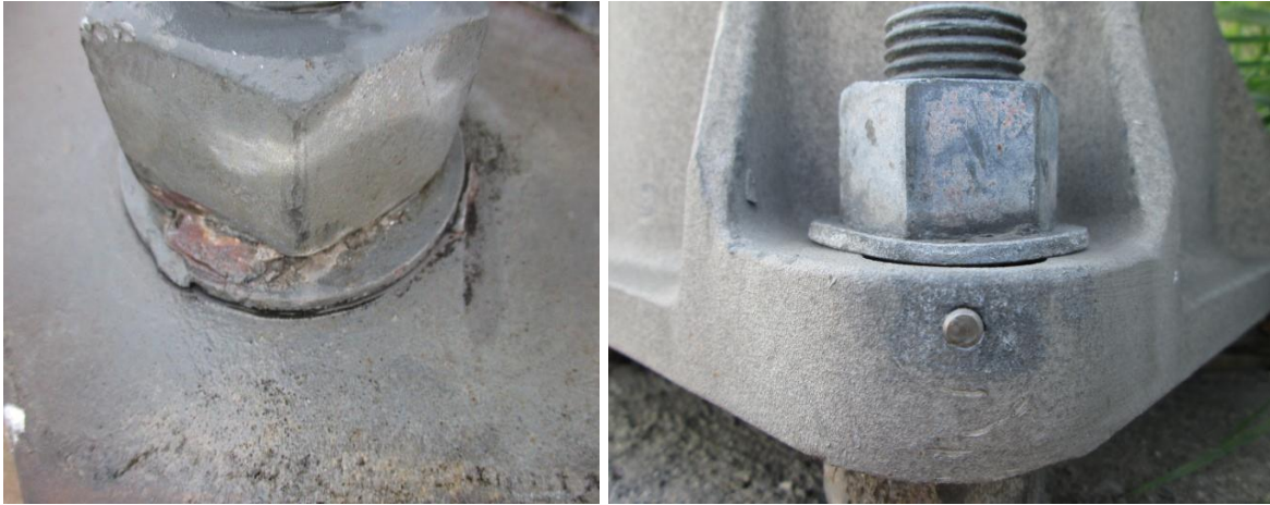
Figure 11-12: Anchor bolt and leveling nuts foundation, nut tack welded to washer (left), incorrect washer type – plate washers intended to cover slotted holes (right)
