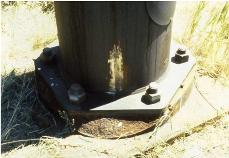
Figure 12-4: HMLT concrete foundation, spalling deterioration
