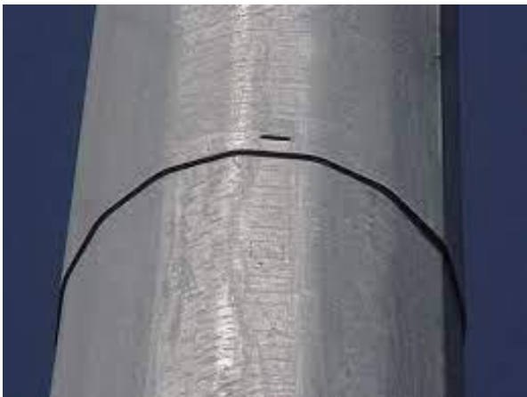
Figure 12-7: HMLT pole splice
