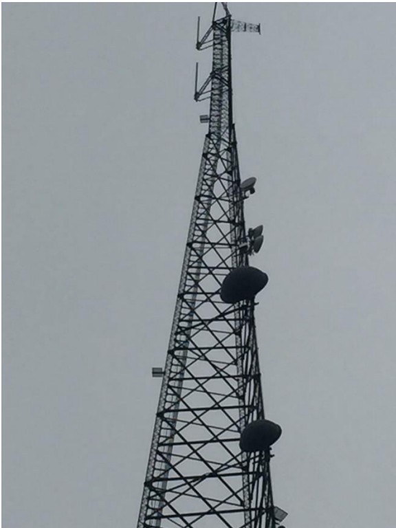
Figure 13-5: Communication tower with vertical supports and diagonal and horizontal bracing
