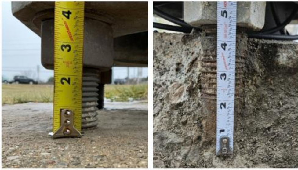
Figure 13-4: Standoff measurement for a sound foundation (left) and standoff measurement with foundation concrete deterioration (right)
