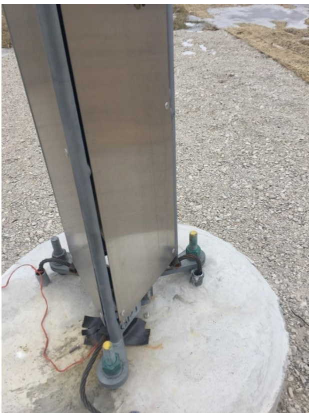
Figure 14-6: ESS tower base plate
