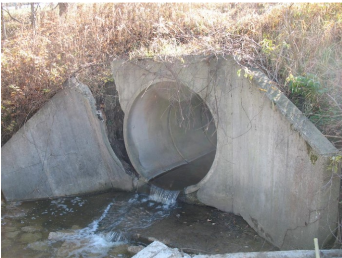
Figure 2-27: Concrete foundation and wingwall damage due to scour
