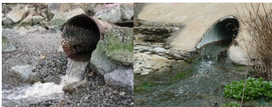
Figure 2-13: Stream channel poor vertical alignment (left) and horizontal alignment (right)
