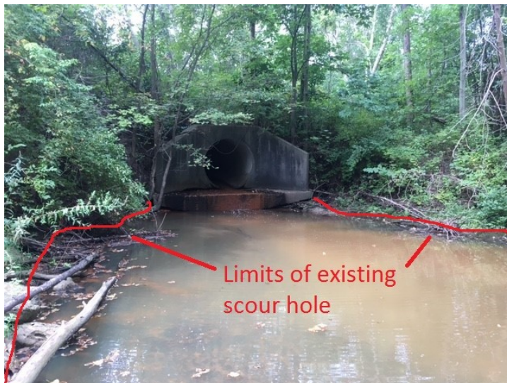
Figure 2-28: Perched outlet with large scour hole
