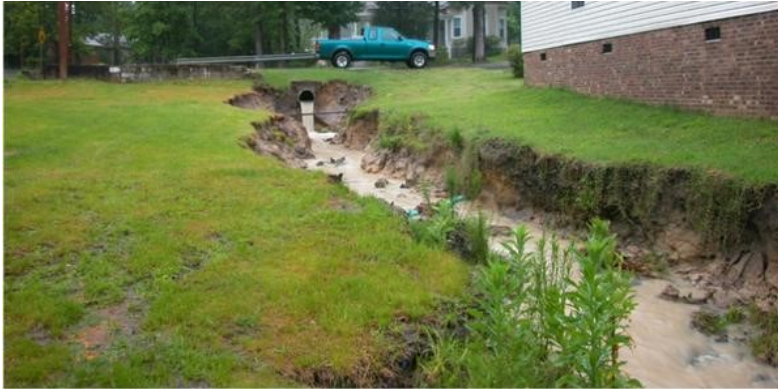
Figure 2-21: No scour (left), scour hole (right)
