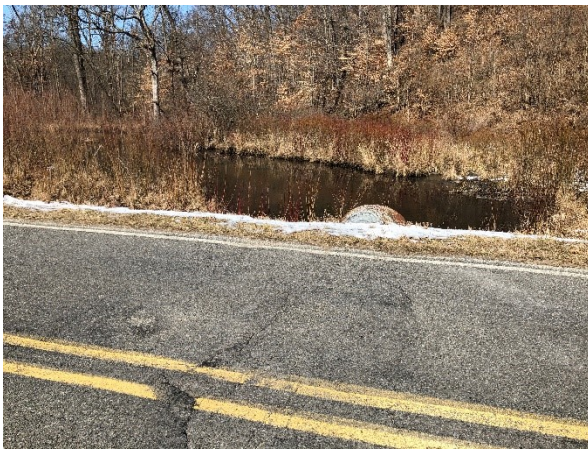
Figure 2-6: Transverse cracking of pavement above culvert
