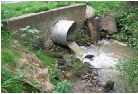
Figure 2-17: Vertical alignment distress; may have progressing washout due to high flow
