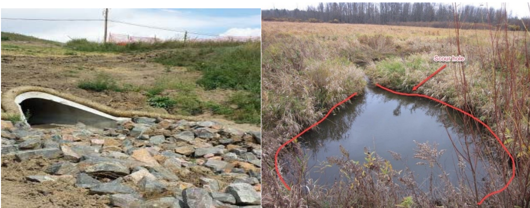
Figure 2-21: No scour (left), scour hole (right)
