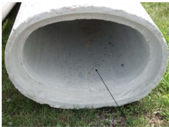
Figure 2-38: Elliptical concrete barrel
