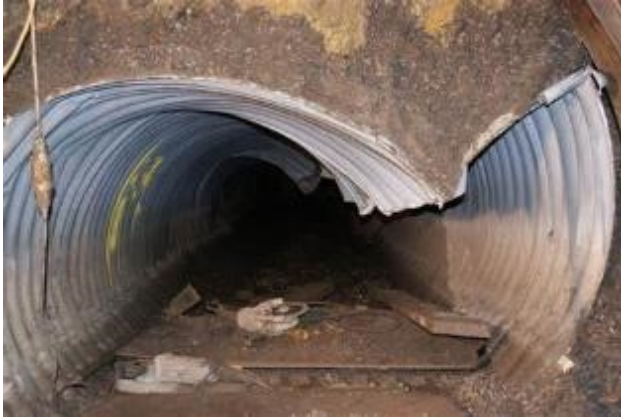
Figure 2-30: Loss of vertical alignment in a corrugated metal culvert
