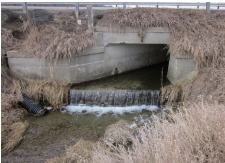
Figure 2-16: Vertical alignment issue leading to stream degradation
