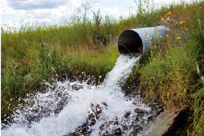
Figure 2-22: Projecting or perched outlet
