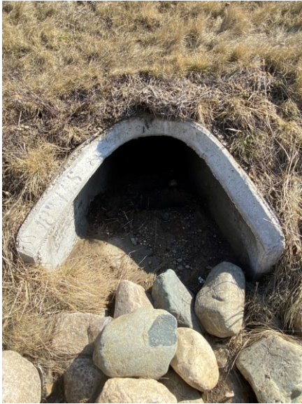
Figure 2-24: Flared concrete end section
