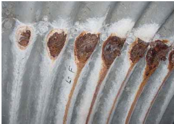
Figure 2-35: Corrosion of a metal culvert
