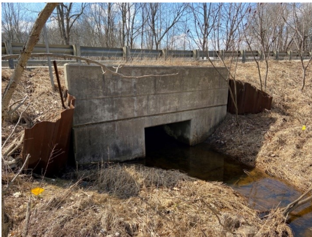
Figure 2-25: Concrete headwall and metal sheet pile wingwalls
