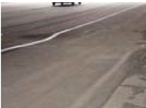
Figure 2-5: Pavement and shoulder issues above culverts
