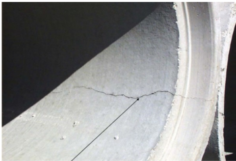
Figure 2-32: Longitudinal crack within a concrete barrel
