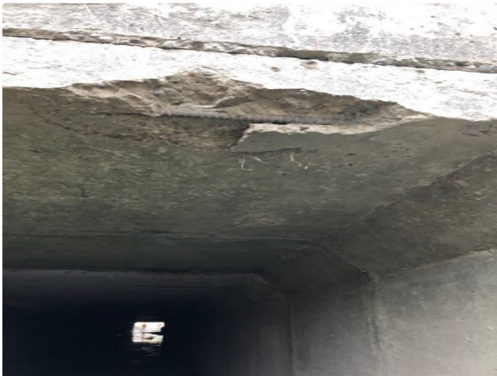
Figure 2-26: Spalled concrete at headwall
