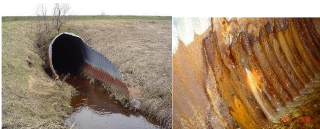
Figure 2-36: Loss of protective coatings contributing to corrosion
