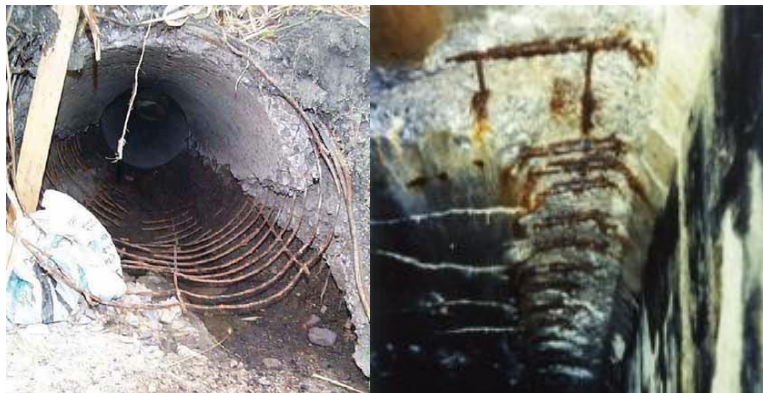
Figure 2-34: Concrete barrel deterioration
