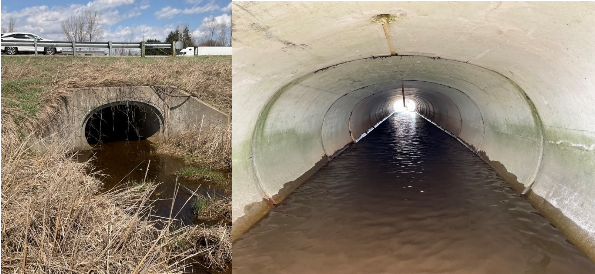
Figure 2-31: Concrete barrel culvert
