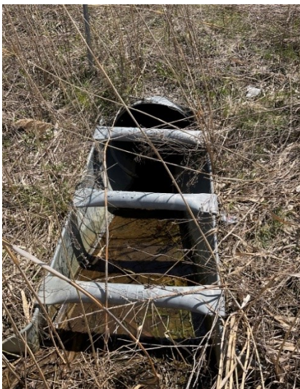
Figure 2-23: Sloped metal end sections
