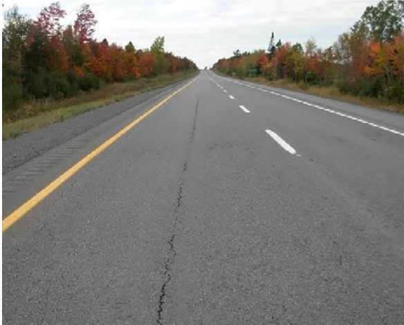
Figure 2-7: Longitudinal cracking
