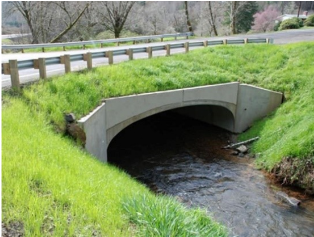
Figure 2-25: Concrete headwall and metal sheet pile wingwalls
