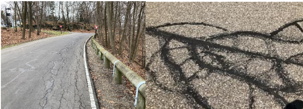
Figure 2-8: Pavement and shoulder alligator cracking
