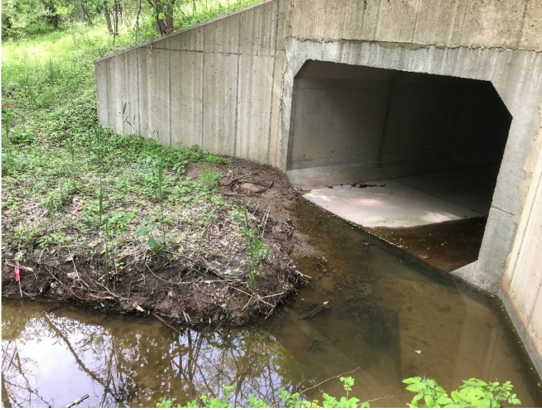
Figure 2-14: Stream channel poor horizontal alignment
