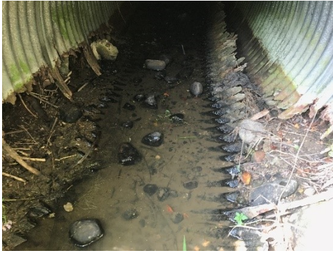
Figure 2-37: Abrasion wearing away corrugated metal pipe corrugations
