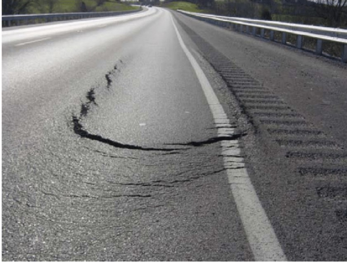
Figure 2-9: Slippage cracking
