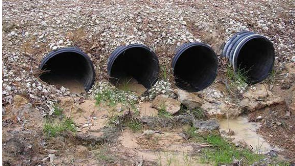
Figure 2-12: Culvert erosion—early-stage gully/rill erosion between the culverts
