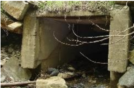
Figure 2-16: Vertical alignment issue leading to stream degradation
