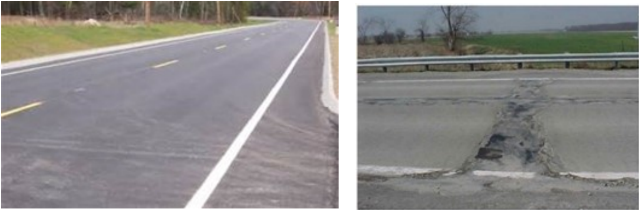
Figure 2-4: Approach roadway, without observable distress (left), clear distress over culvert (right)
