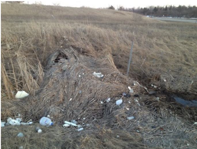
Figure 2-18: Blocked inlet
