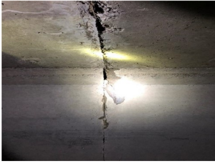
Figure 2-33: Spalling within a box culvert
