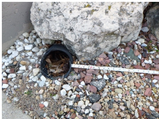
Figure 3-43: Drainage outlet is partially clogged with leaves and debris
