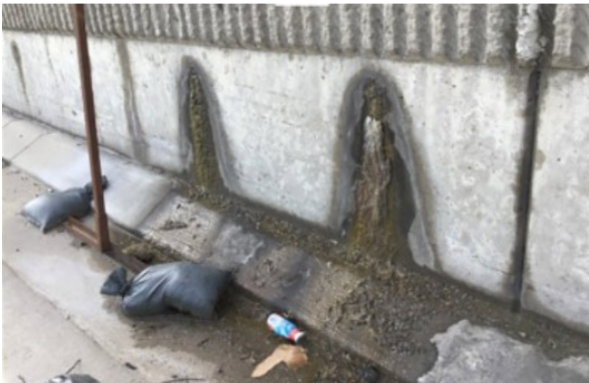
Figure 3-13: Retaining wall concrete abrasion
