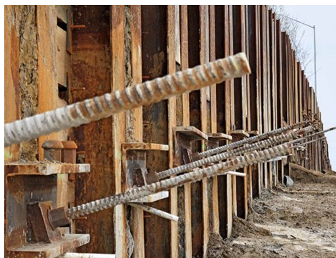
Figure 3-37: Wall anchor
