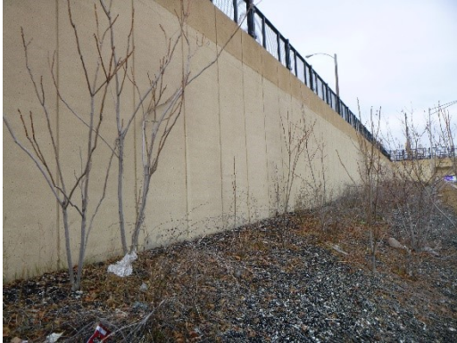
Figure 3-14: Semi-protective concrete protective coating
