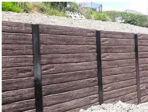
Figure 3-38: Vertical support steel
