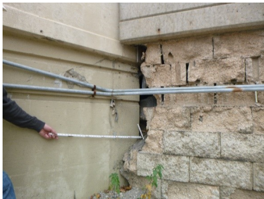
Figure 3-24: Masonry breakdown
