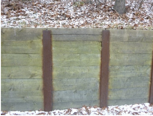
Figure 3-21: Timber lagging is split along top
