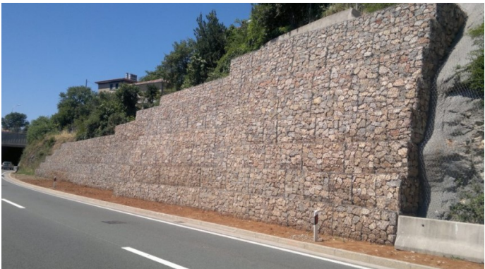
Figure 3-34: Gabion wall
