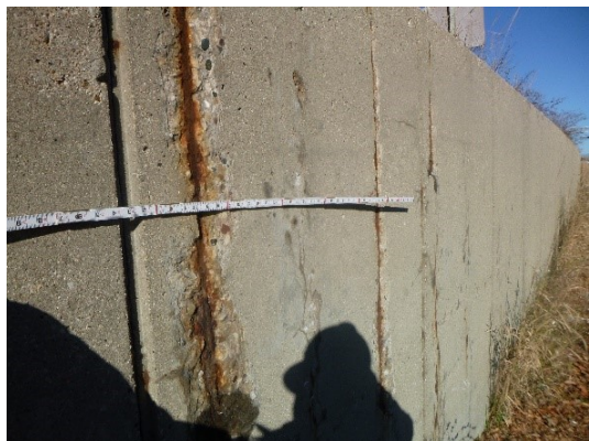
Figure 3-10: Corroded wall reinforcing
