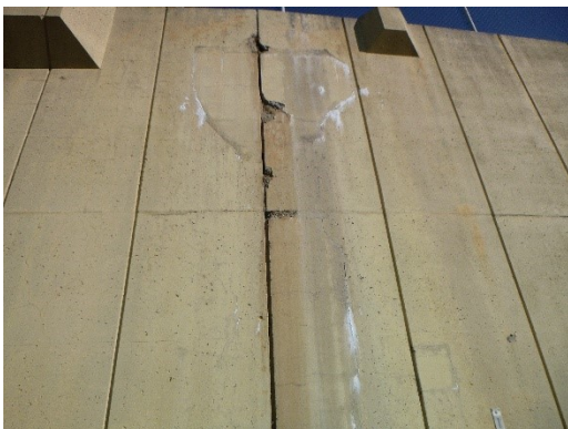
Figure 3-15: Efflorescence accumulation
