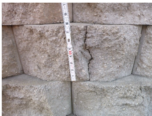
Figure 3-23: Vertical split in modular block
