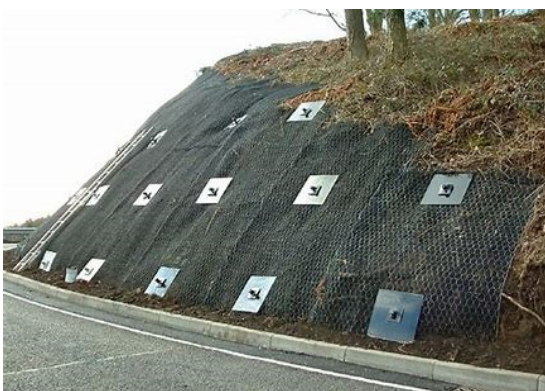
Figure 3-32: Typical soil nail wall
