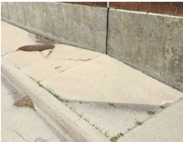
Figure 3-42: Wall settlement
