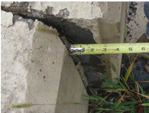
Figure 3-36: Wall displacement
