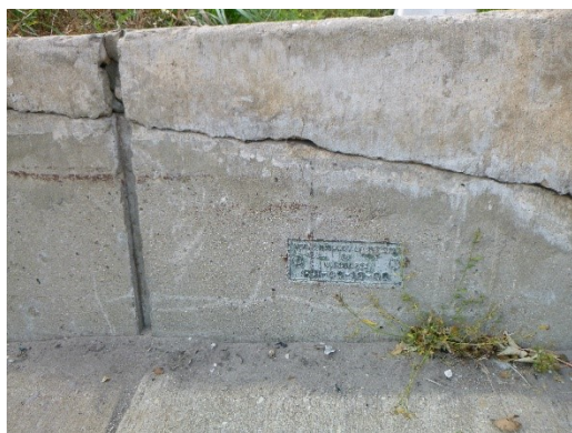
Figure 3-9: Horizontal structural cracking
