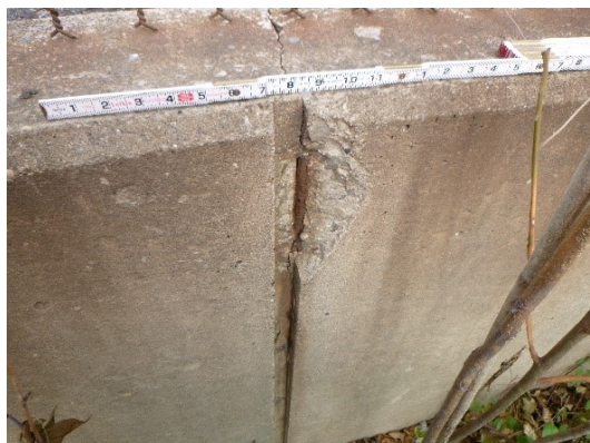
Figure 3-11: Concrete spall with corroded reinforcing
