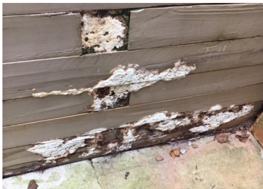
Figure 3-20: Timber lagging splitting
