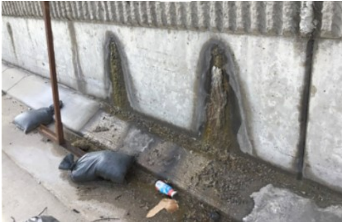
Figure 3-16: Weep holes/wall drainage
