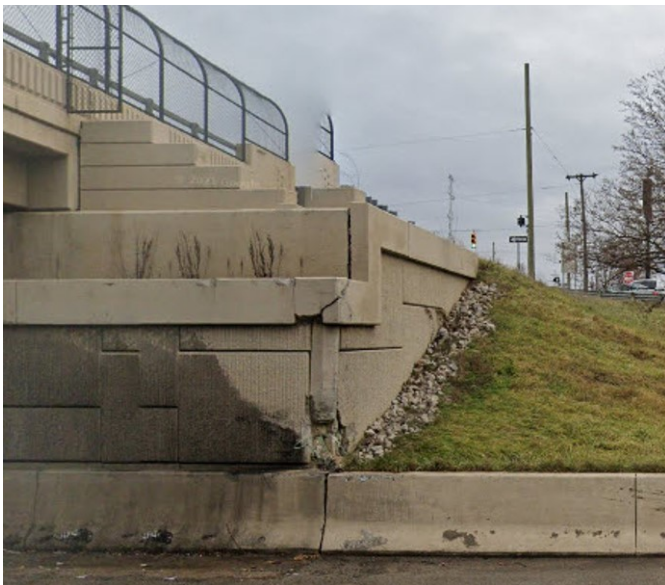
Figure 3-17: Impact damage
