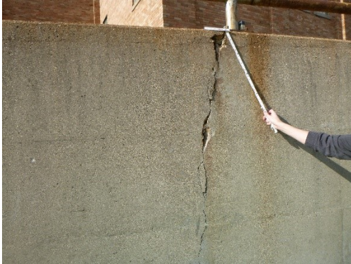
Figure 3-12: Spalled and delaminated concrete
