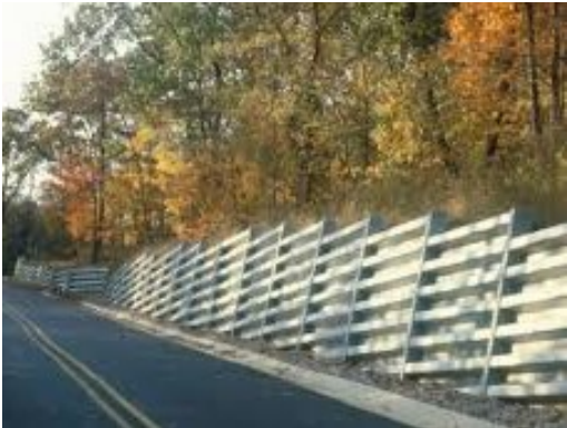
Figure 3-27: Typical metal bin wall
