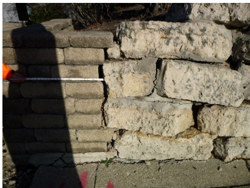
Figure 3-25: Wall misalignment
