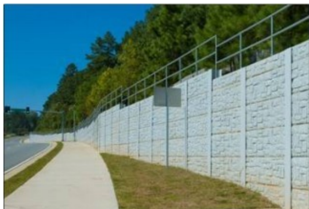
Figure 3-30: Soldier pile wall with precast lagging (note: anchors not shown)
