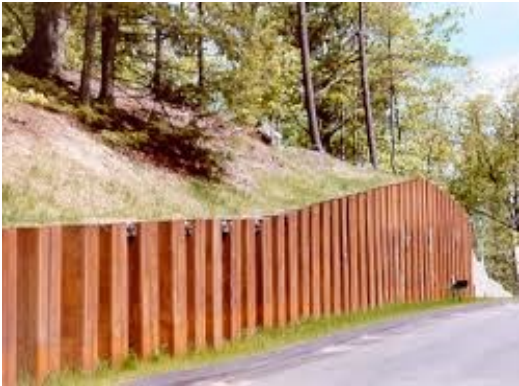
Figure 3-27: Typical metal bin wall
