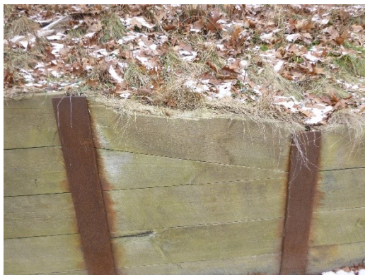
Figure 3-20: Timber lagging splitting
