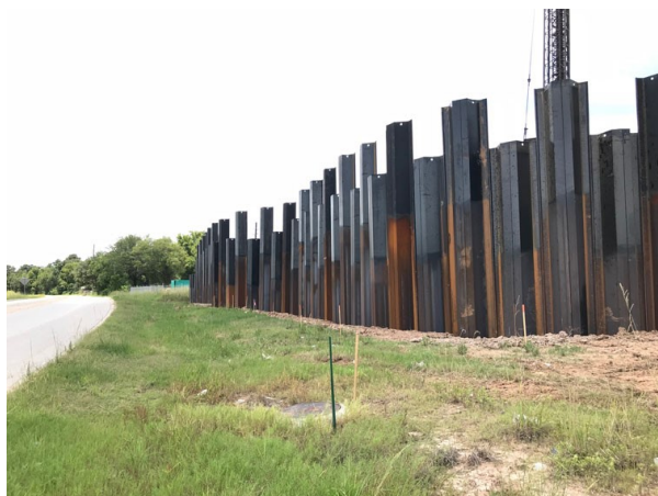
Figure 3-29: Steel protective coating missing
