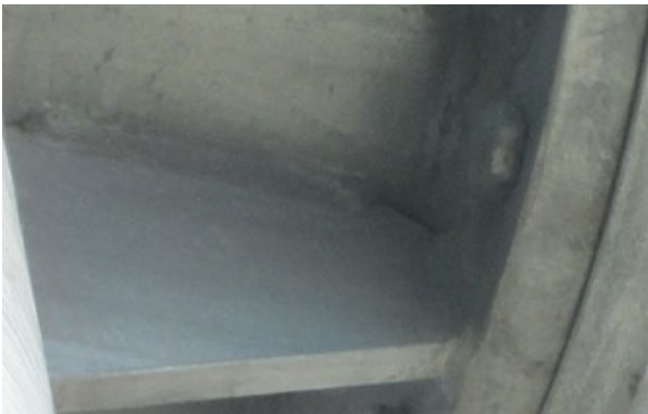
Figure 4-13: Vertical structure connection, missing flat washer on head side of bolt
