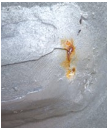
Figure 4-15: Vertical structure connection, rust bleeding through galvanizing at welded gusset plate arm to vertical structure upright
