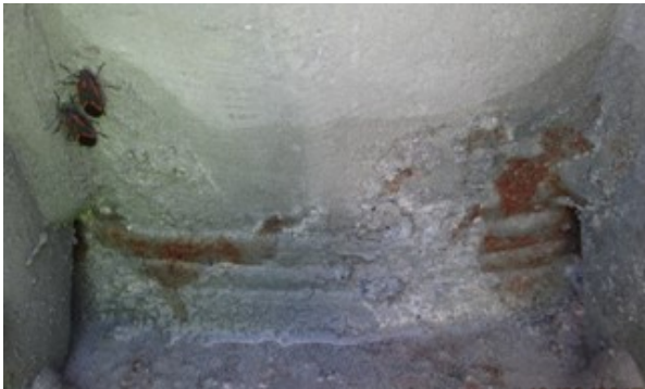
Figure 4-11: Cantilever or truss structure base plate and vertical support, rust underneath galvanizing repair
