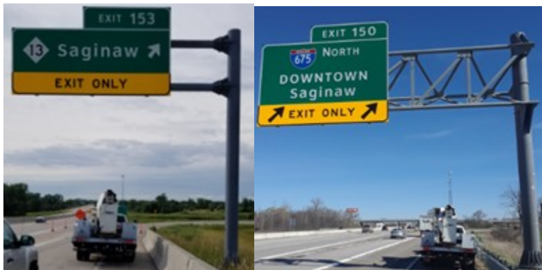
Figure 4-1: Cantilever structure, two-arm (left) and tri-chord style (right)
