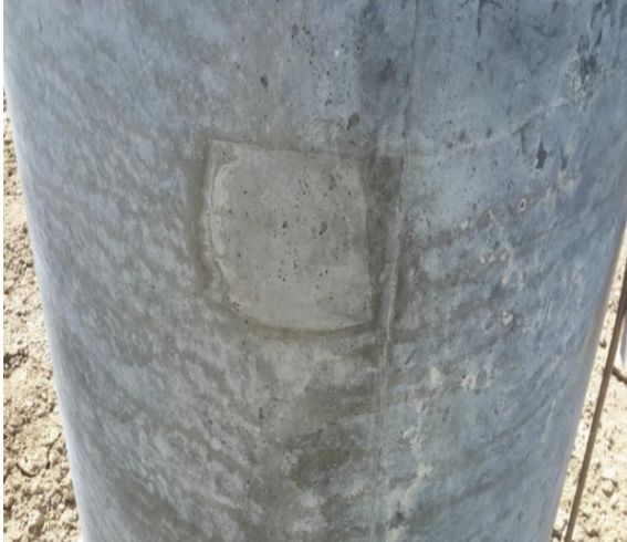
Figure 6-5: Crack with rusted rebar water leakage
