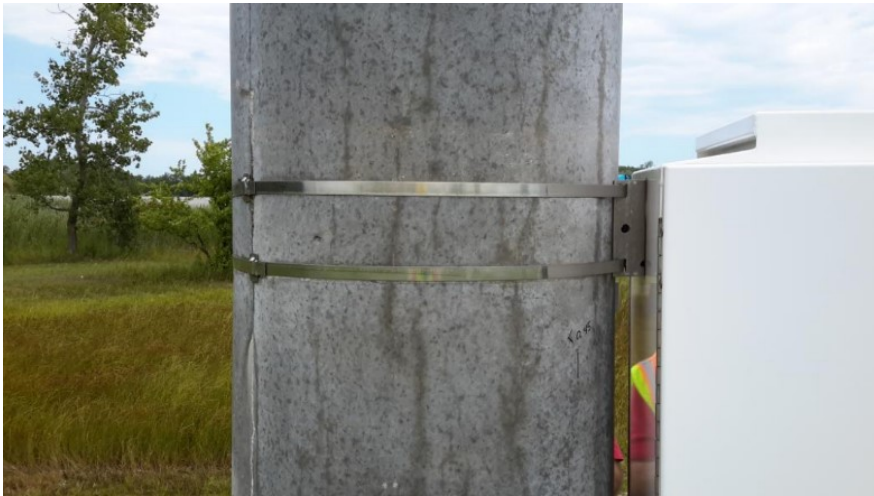
Figure 6-7: Band clamp connection to metal enclosure
