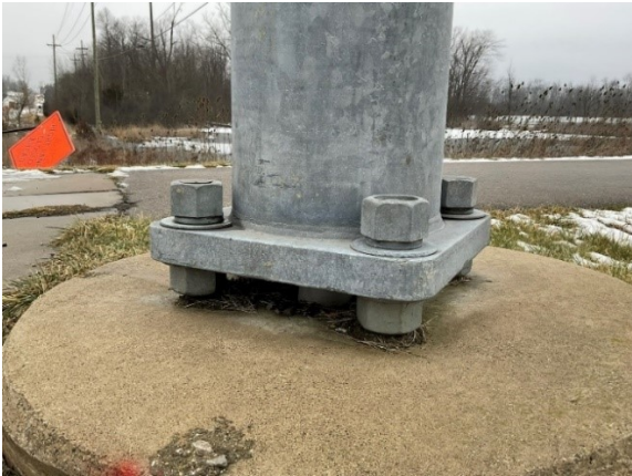
Figure 7-10: Steel strain pole foundation with excess standoff distance and nut covers
