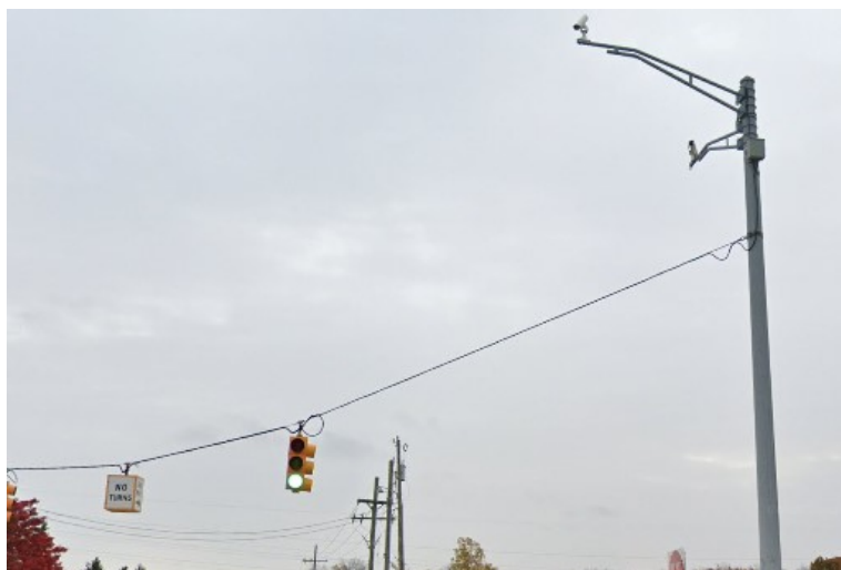
Figure 7-20: Cameras mounted on luminaire truss arms
