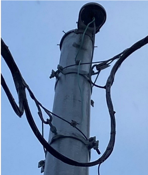
Figure 7-14: Steel strain pole bracket assembly connections for luminaire arms
