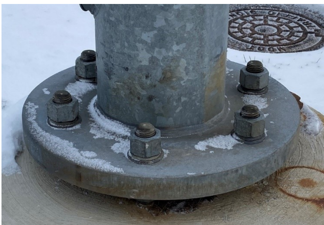
Figure 7-11: Steel strain pole base plate with six anchor bolts
