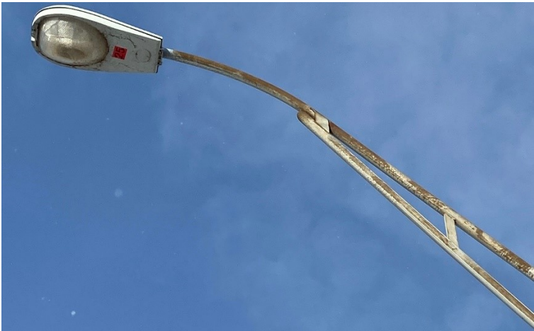
Figure 7-19: Luminaire and luminaire truss arm
