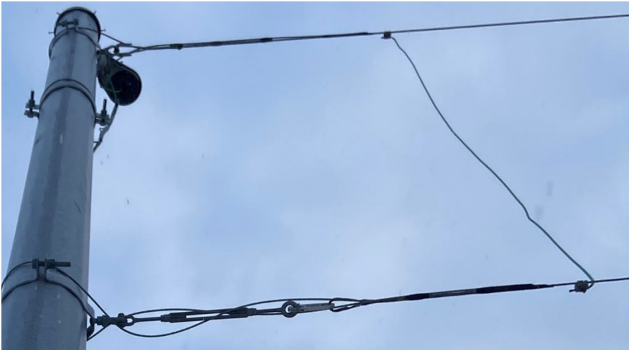
Figure 7-16: Span wire assemblies attached to steel strain pole band clamps
