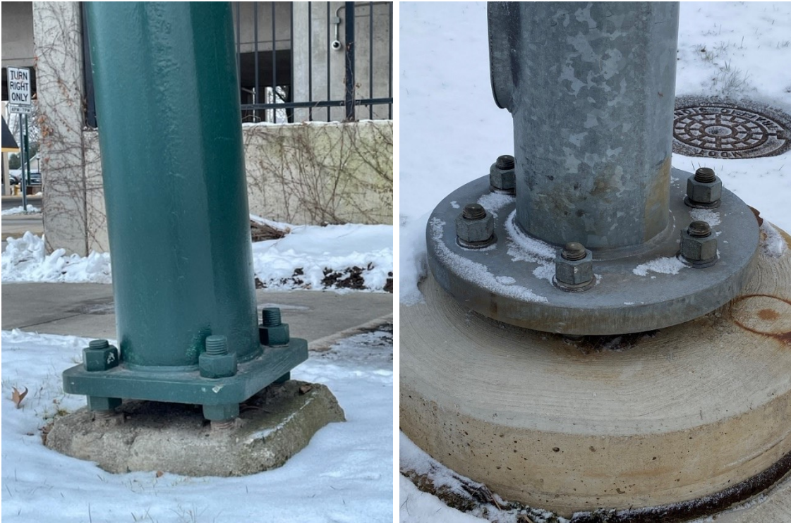
Figure 7-7: Steel strain pole square foundation with four anchor bolts (left, note misalignment), newer style drilled shaft foundation with six anchor bolts (right)
