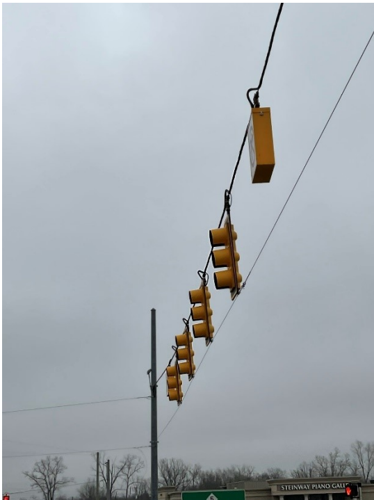
Figure 7-15: Steel strain pole span wire supporting signals and sign
