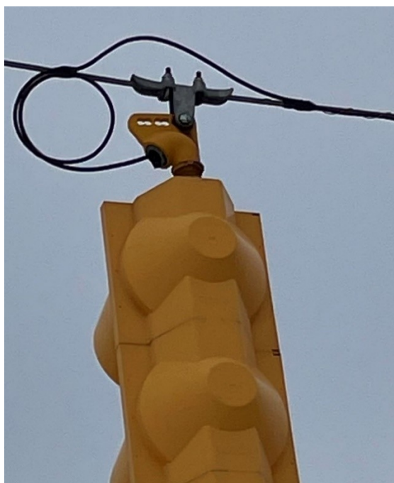
Figure 7-18: Span wire hanger
