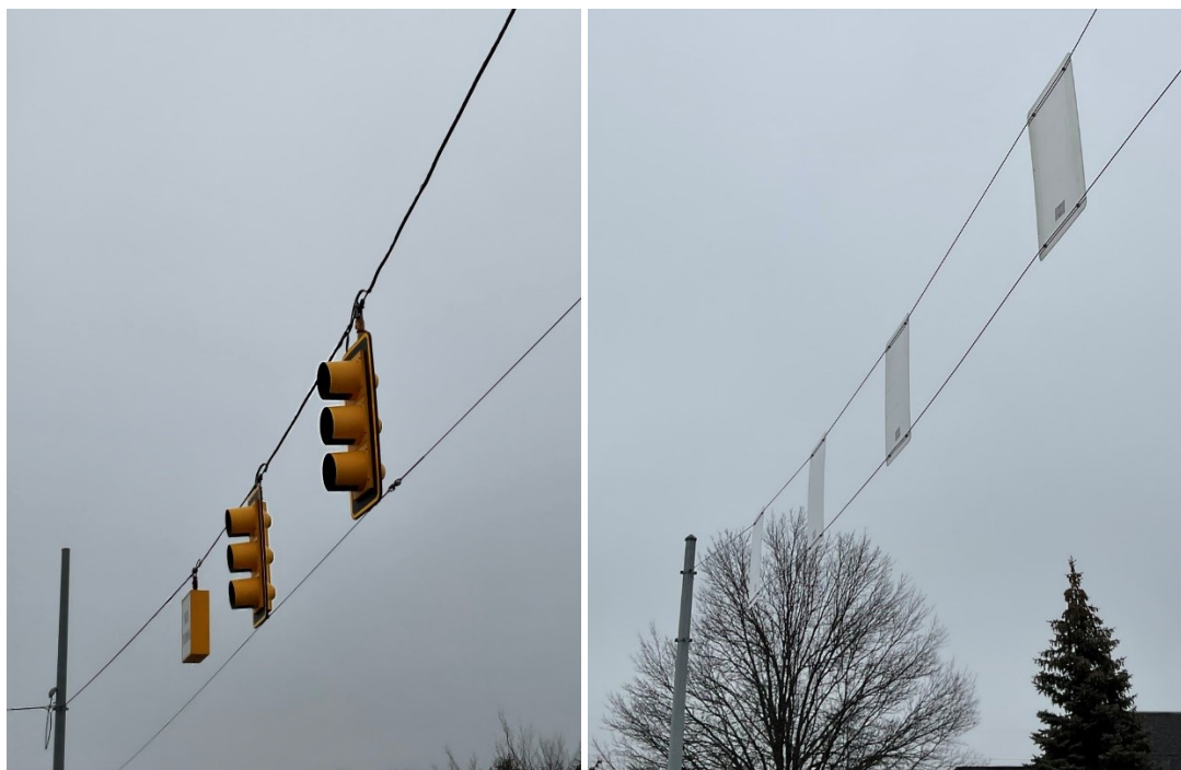
Figure 7-18: Span wire hanger
