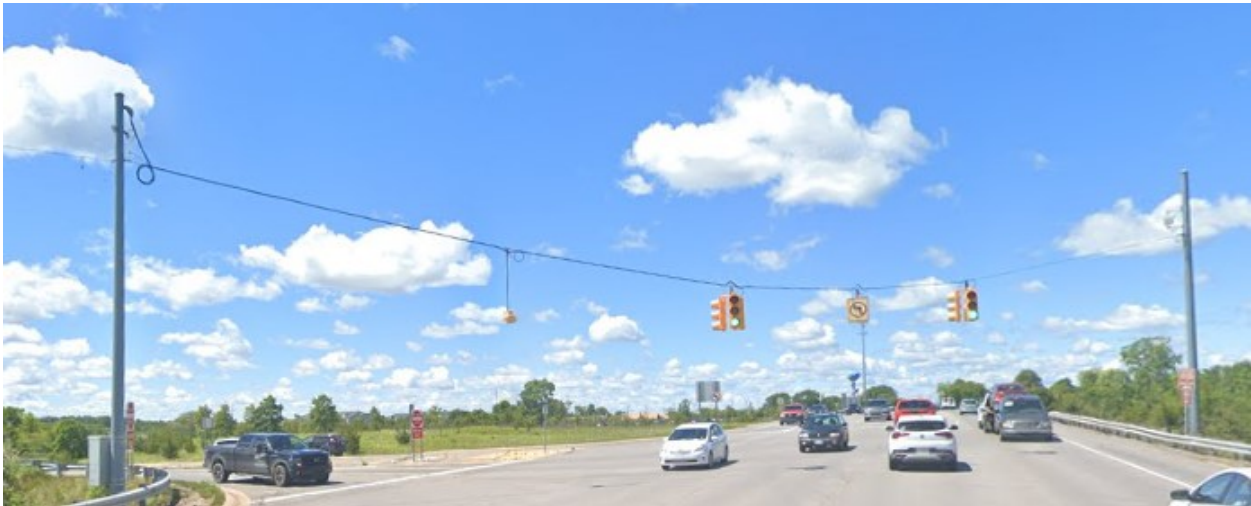
Figure 7-4: Steel strain poles with single diagonal span configuration
