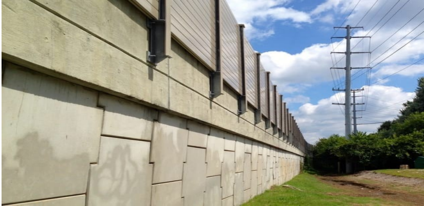
Figure 8-5: Noise wall attached to retaining wall
