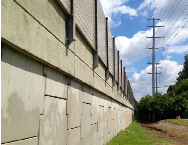
Figure 8-11: Noise wall attached to retaining wall
