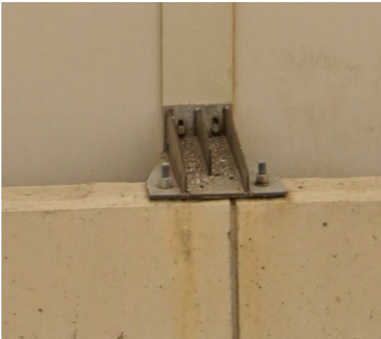
Figure 8-10: Noise wall attachment to concrete barrier
