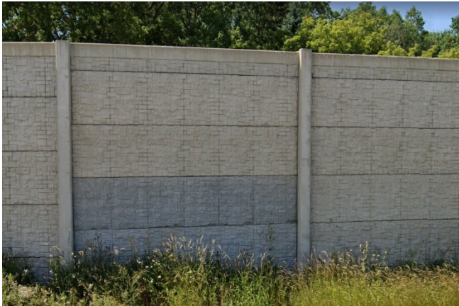
Figure 8-9: Noise Wall with masonry block indicating T-wall joint element
