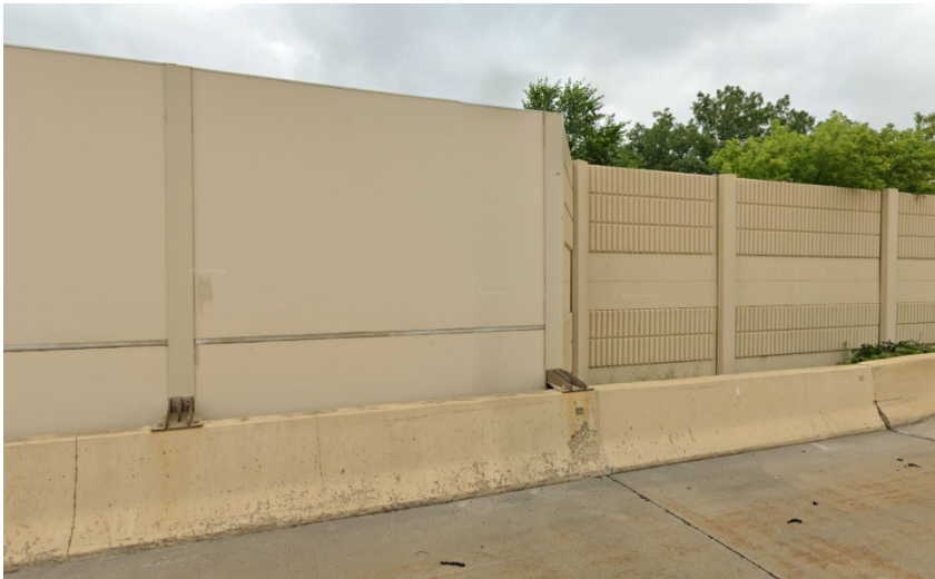
Figure 8-4: Noise wall mounted on crash barrier
