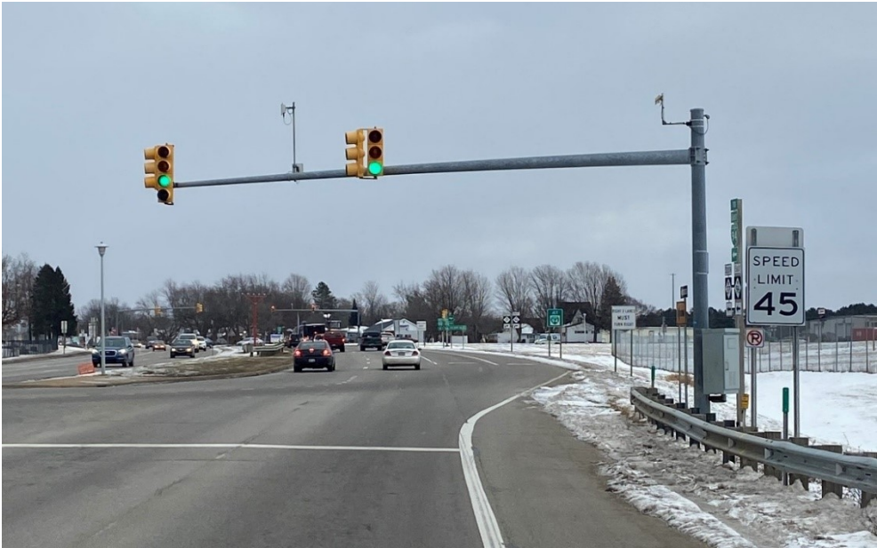
Figure 9-14: Mast arm structure with single arm
