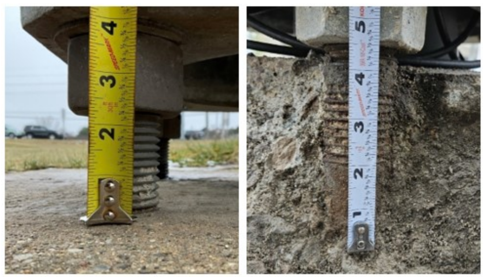
Figure 9-7: Standoff measurement for a sound foundation (left) and standoff measurement with foundation concrete deterioration (right)
