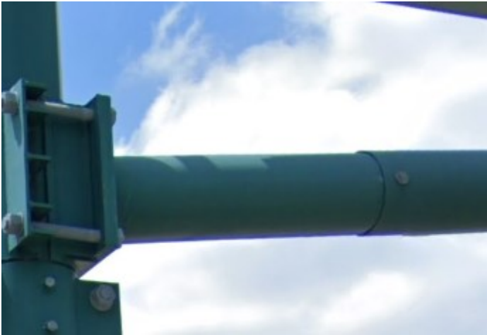
Figure 9-15: Mast arm member splice with connection bolt
