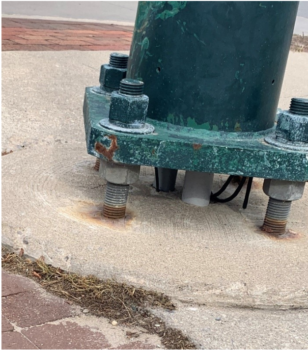
Figure 9-8: Four anchor bolt foundation with excessive standoff distance and corrosion
