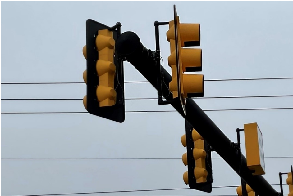
Figure 9-16: Mast arm signal and sign attachment connections
