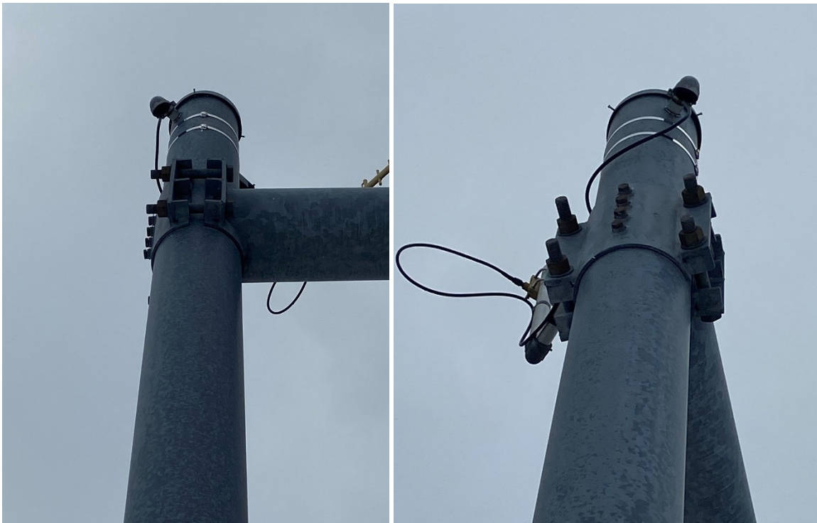
Figure 9-11: Mast arm to pole vertical structure connection, saddle clamp type
