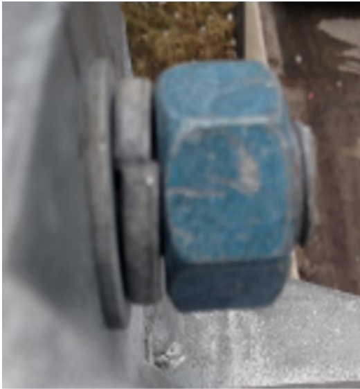
Figure 10-13: Vertical structure connection, loose bolt/lock washer not fully compressed
