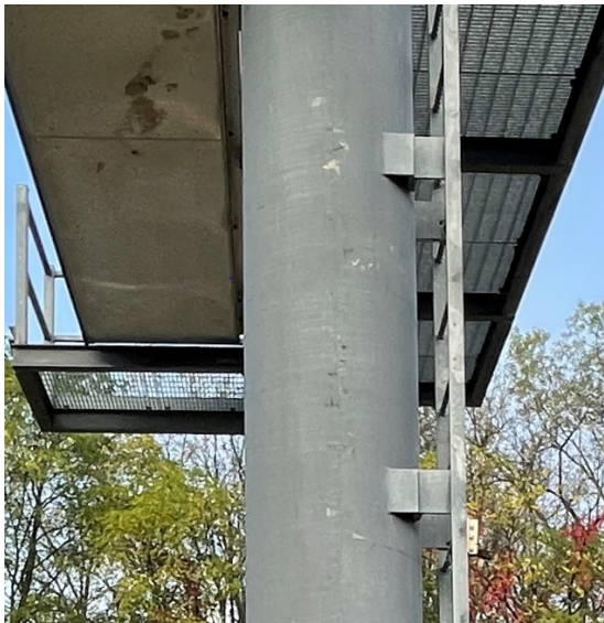
Figure 10-11: Vertical structure column (upright) with minor coating damage
