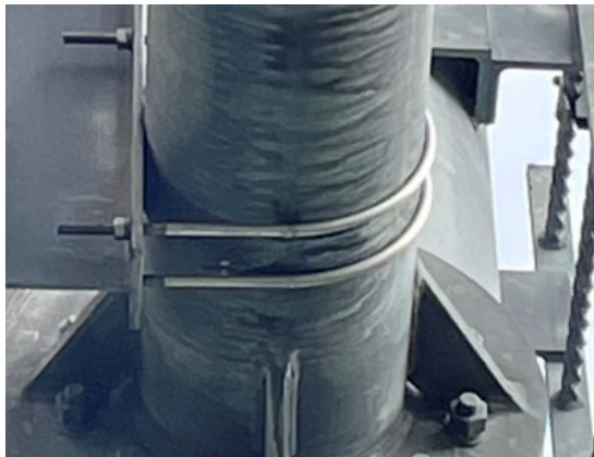
Figure 10-16: Horizontal structure connection, broken U-bolt connection at the nut end
