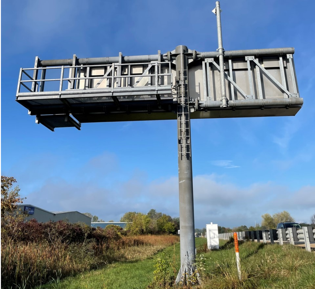
Figure 10-3: Dynamic Message Sign Support Structure
