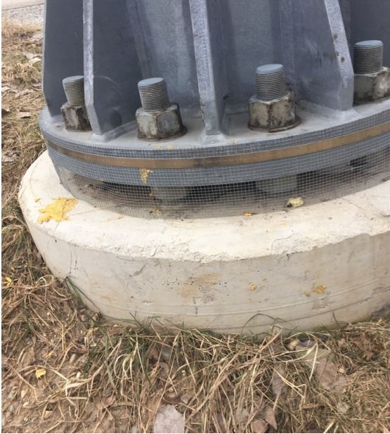
Figure 10-4: DMS support structure foundation, minor spalling
