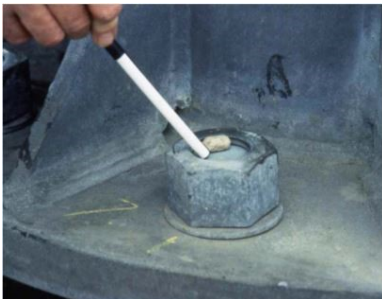
Figure 10-8: Leveling nut and anchor bolt corrosion with section loss
