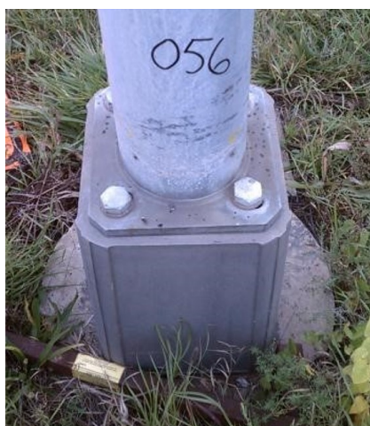
Figure 11-14: Frangible base connections, exposed bolt hole
