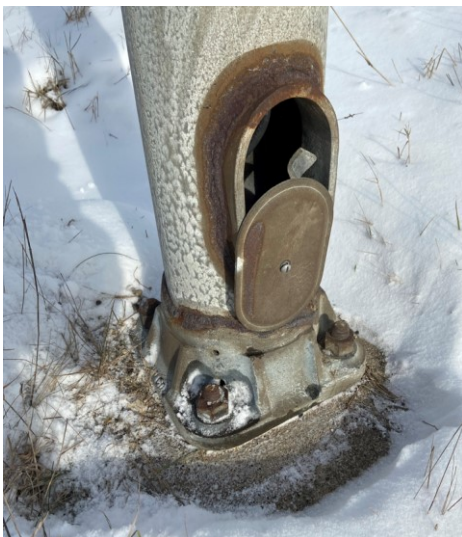
Figure 11-20: Non-frangible pole structure vertical support column (upright), loosely covered handhole
