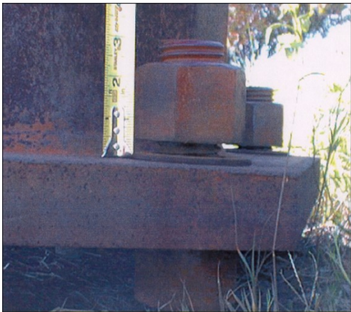
Figure 11-11: Anchor bolt and leveling nut foundation, gap between anchor nut and washer in corroding base unit (left), gap between anchor nut and washer with bolt out of plumb and debris between upright base and concrete foundation (right)
