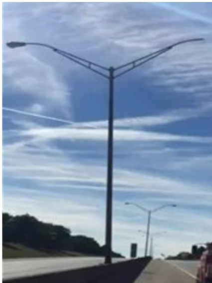
Figure 11-24: Luminaire and luminaire arm element, missing luminaire head
