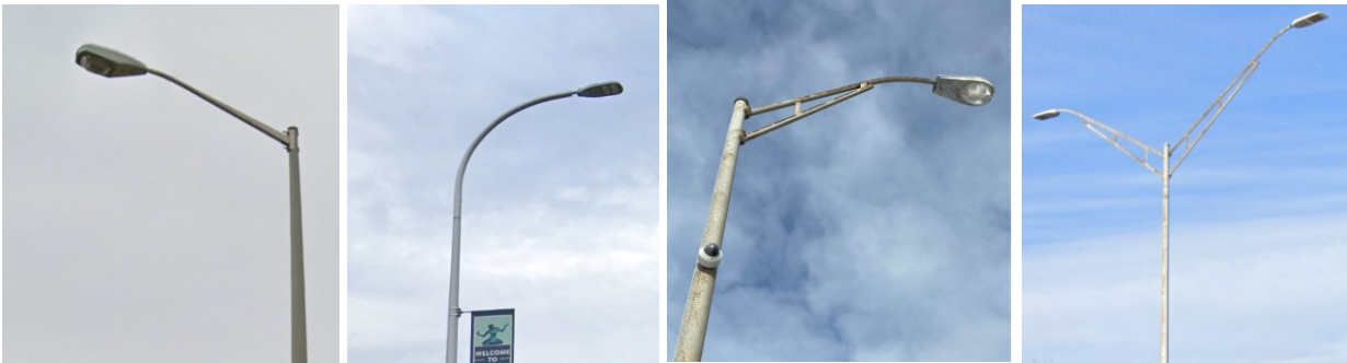
Figure 11-1: Pole structure arm types (numbering from left), single member (1), Davit member (2), single truss arm (3), double truss arm member (4)
