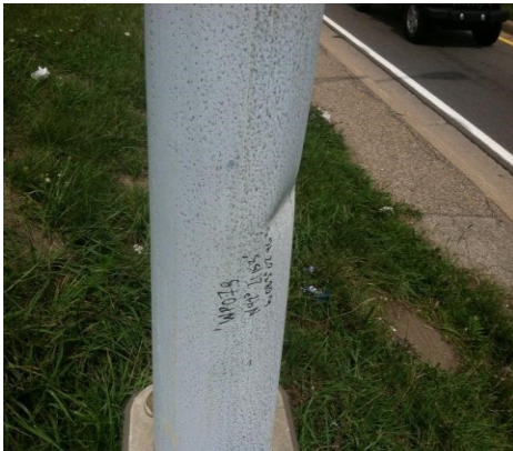
Figure 11-20: Non-frangible pole structure vertical support column (upright), loosely covered handhole
