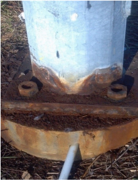
Figure 11-17: Base plate, pole corrosion and section loss at base weld
