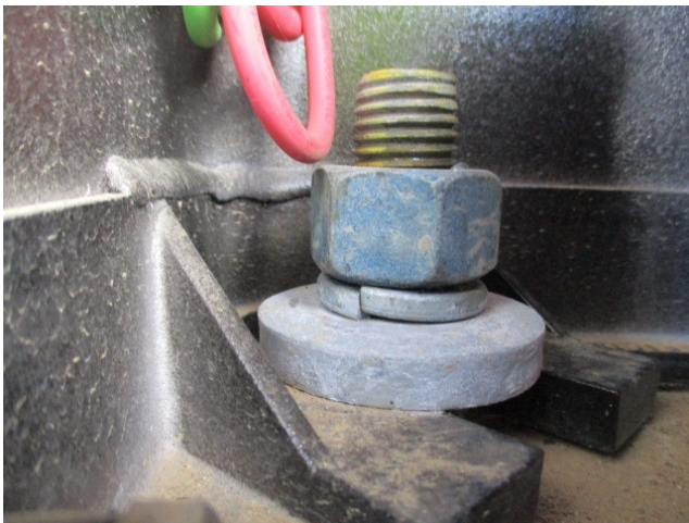
Figure 11-9: Frangible pole structure anchor bolts and leveling nuts foundation, loose anchor bolt (left), anchor nut without fully engaged thread (right)
