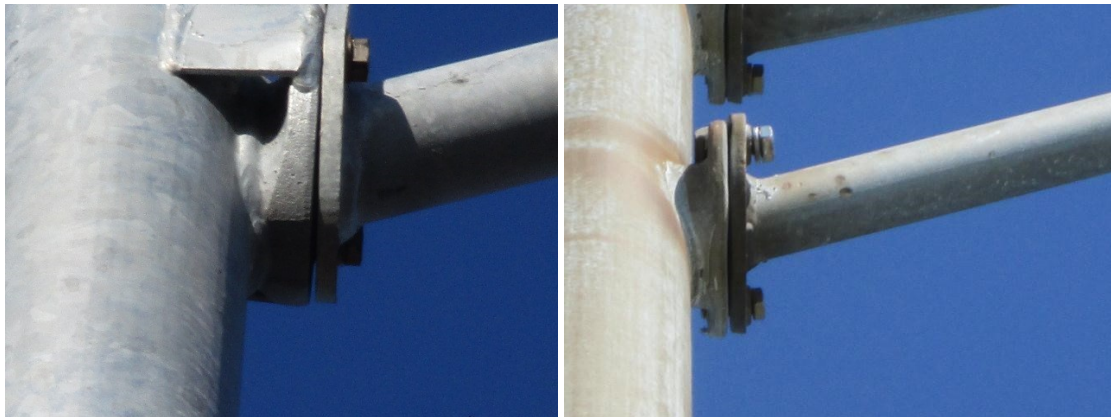
Figure 11-22: Frangible and non-frangible pole structure vertical structure connections, gap at arm flange (left), loose arm connection bolt (right)
