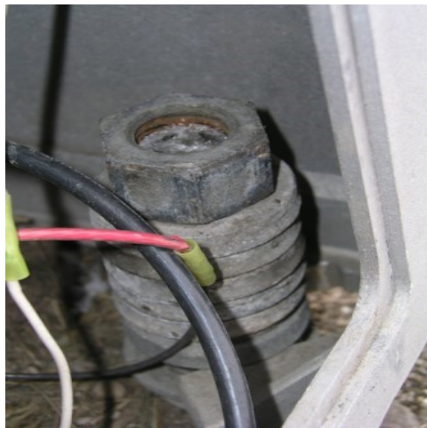
Figure 11-9: Frangible pole structure anchor bolts and leveling nuts foundation, loose anchor bolt (left), anchor nut without fully engaged thread (right)
