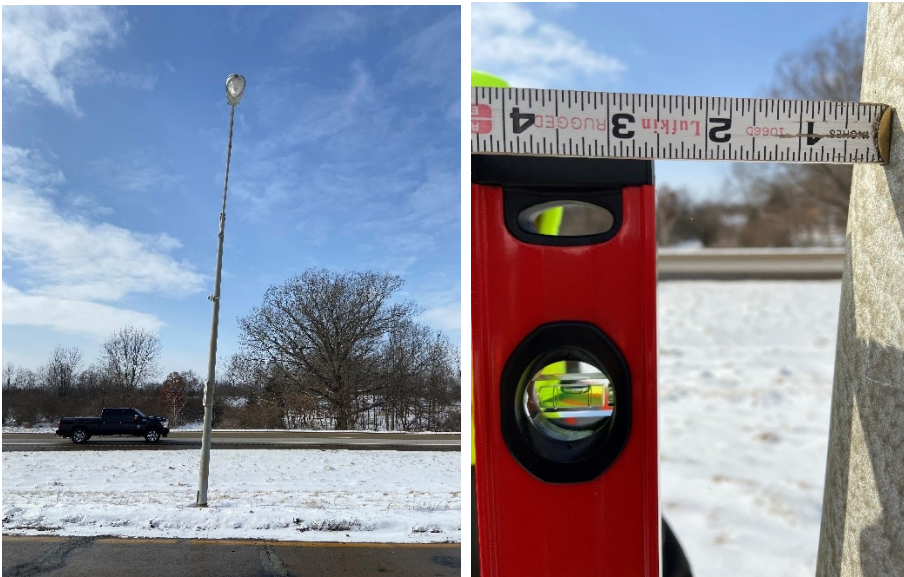
Figure 11-21: Non-frangible pole structure vertical support column (upright), visual identification of out of plumb pole (left), measurement of pole plumbness (right)
