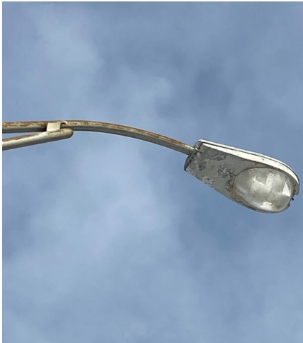
Figure 11-23: Luminaire and luminaire arm element, evidence of galvanizing damage
