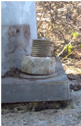
Figure 11-11: Anchor bolt and leveling nut foundation, gap between anchor nut and washer in corroding base unit (left), gap between anchor nut and washer with bolt out of plumb and debris between upright base and concrete foundation (right)
