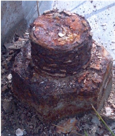
Figure 11-11: Anchor bolt and leveling nut foundation, gap between anchor nut and washer in corroding base unit (left), gap between anchor nut and washer with bolt out of plumb and debris between upright base and concrete foundation (right)
