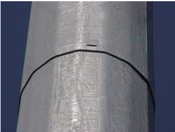
Figure 12-7: HMLT pole splice
