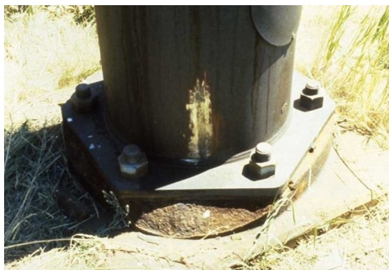
Figure 12-4: HMLT concrete foundation, spalling deterioration
