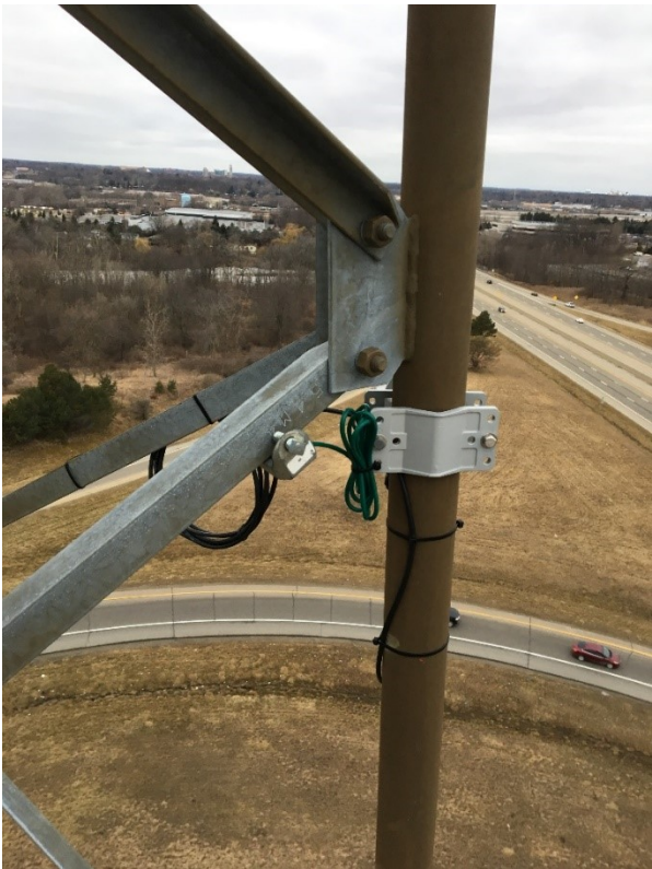
Figure 13-6: Bracing showing vertical structure bolted connection to vertical support
