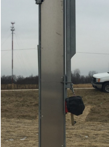
Figure 14-8: ESS tower lowering boom element
