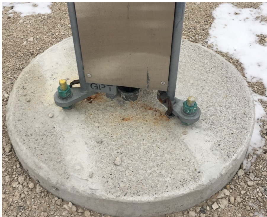
Figure 14-4: ESS tower foundation with triangular anchor bolt pattern
