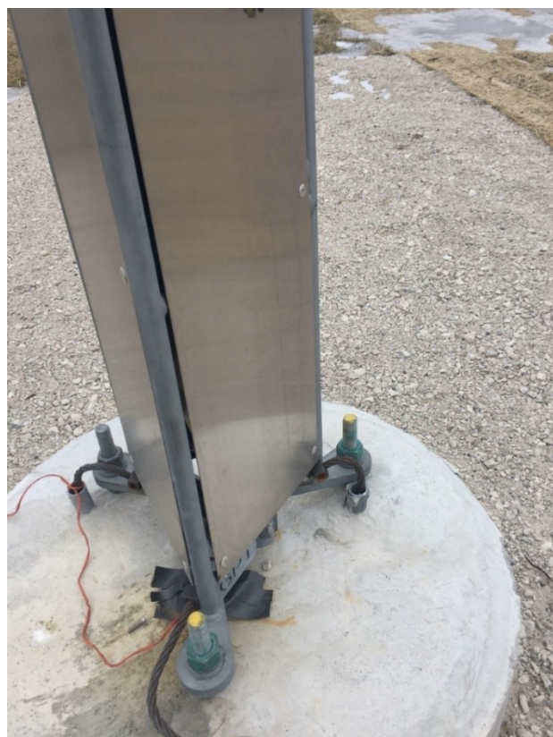
Figure 14-6: ESS tower base plate
