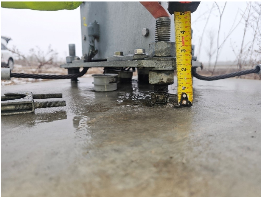
Figure 14-5: Standoff measurement for a sound foundation
