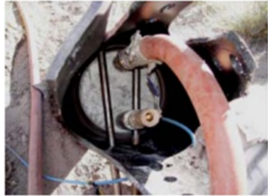
Figure 15: Deform-Reform Liner: Winching Liner (left) and Steam Pressure to Re-round HDPE Liner (right)
