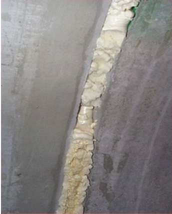
Figure 1: Internal Side of a Chemically Grouted RCP
