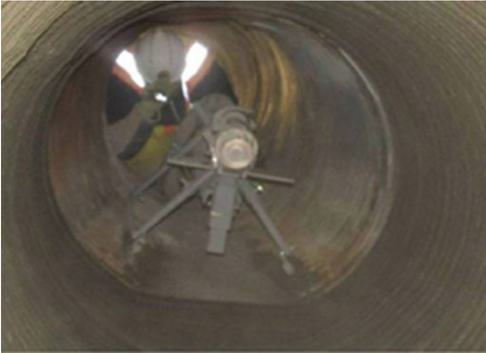
Figure 18: Installation of Centrifugally Cast Liner
