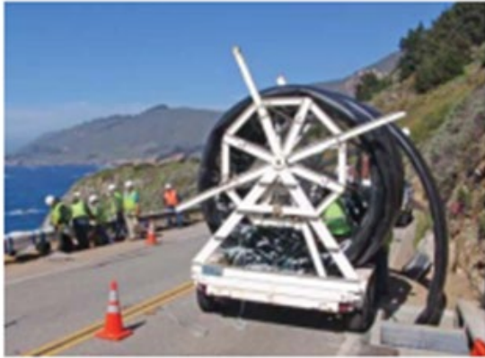
Figure 15: Deform-Reform Liner: Winching Liner (left) and Steam Pressure to Re-round HDPE Liner (right)
