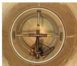
Figure 6: Mechanical Repair Sleeve: PVC Sleeve (left), Two Hydraulic Jacks to Expand Sleeve (middle), and Annular Space Grouting (right)
