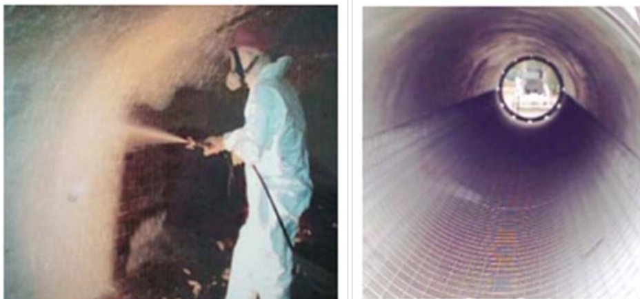
Figure 20: Sprayed-on Liners: Spray Gun Application (left) and Wire Mesh Installation (right)
