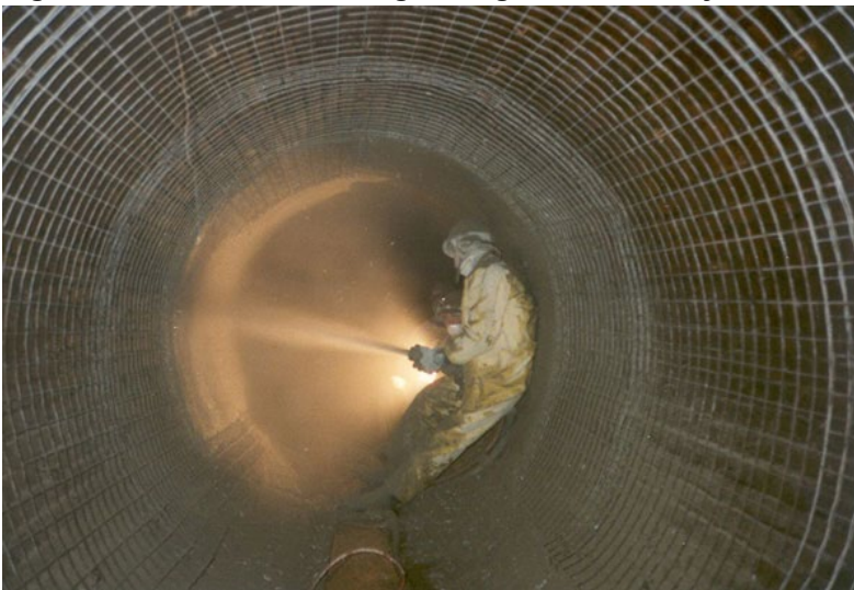
Figure 4: Internal Shotcreting through Human Entry
