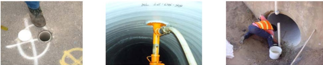
Figure 9: Spirally Wound Liner: Surface Grouting (left), Grouting Through Liner (middle) and Grouting Through Bulkhead (right)
