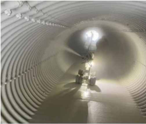
Figure 21: Sprayed-on Liners: Polyurea Coating Application (left) and Robotic Liner System (right)
