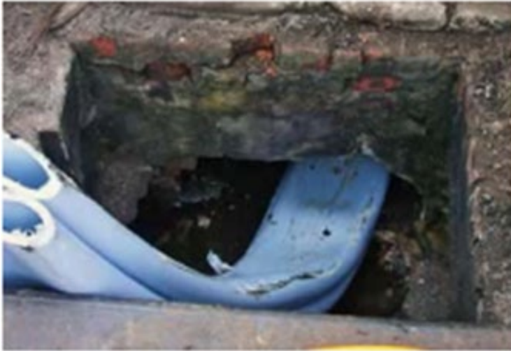
Figure 12: Fold-and-Form Liner: Liner Protruding (left) and Steam Pressure to Re-round PVC Liner (right)
