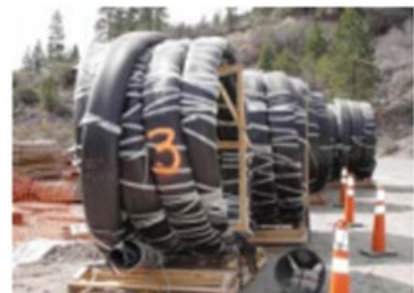
Figure 14: Deform-Reform Liner: "Heart" Shape of Folded HDPE Liner (left), Plastic Bands to Maintain the Shape (middle), and Coiled Pipe to Transport (right)
