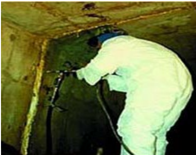
Figure 2: Internal Grouting through Human Entry
