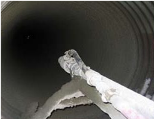
Figure 5: Robotic Shotcreting
