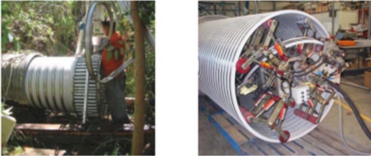
Figure 8: Spirally Wound Liner: Stationary (left) and Mobile (right) Winding Machines
