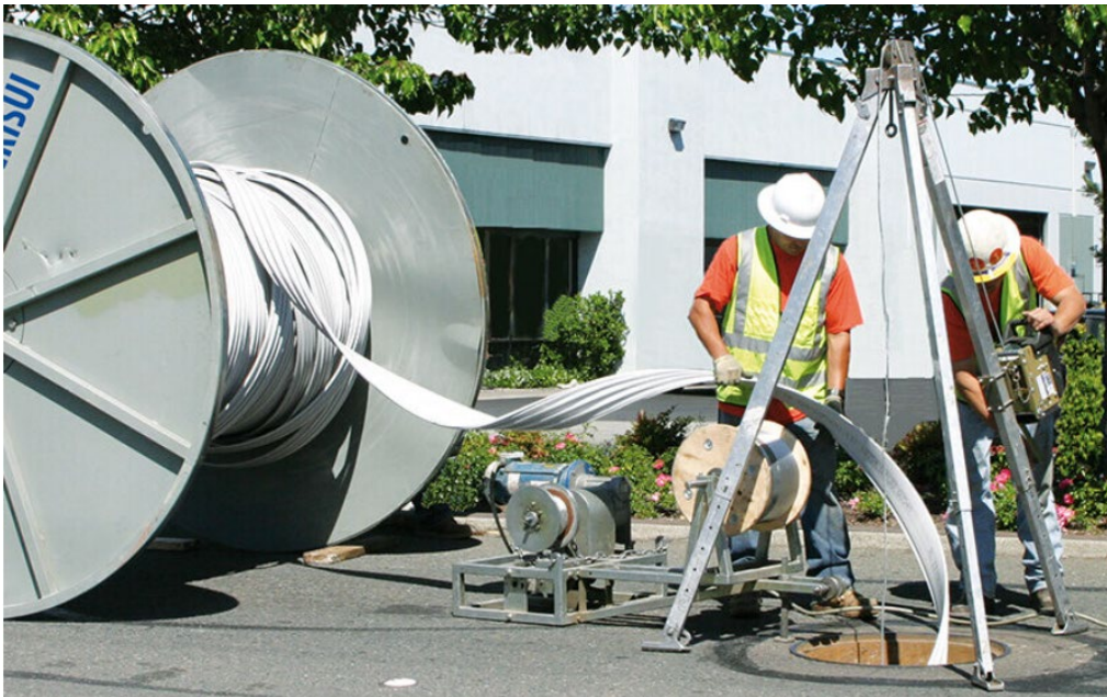
Figure 10: Spiral-wound Lining
