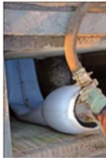
Figure 12: Fold-and-Form Liner: Liner Protruding (left) and Steam Pressure to Re-round PVC Liner (right)
