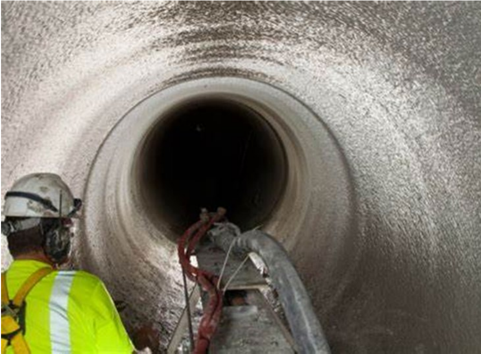
Figure 17: Centrifugally Cast Concrete Pipe Lining
