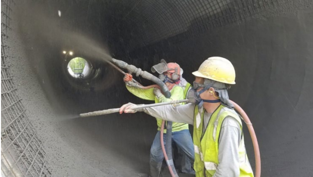
Figure 25: Shotcrete Lining
