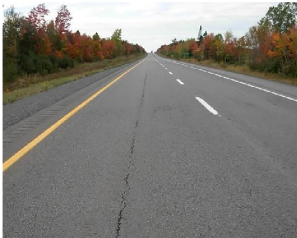
Figure 2-7: Longitudinal cracking
