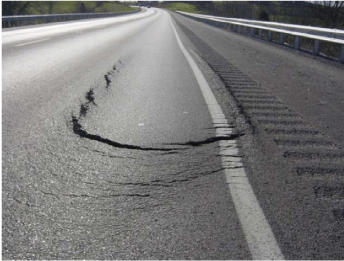
Figure 2-9: Slippage cracking
