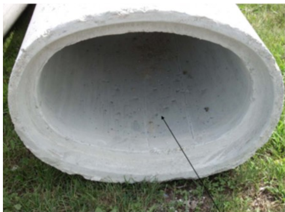
Figure 2-38: Elliptical concrete barrel
