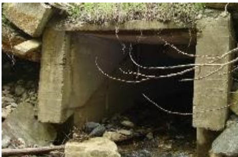
Figure 2-16: Vertical alignment issue leading to stream degradation
