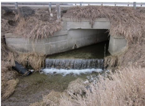
Figure 2-16: Vertical alignment issue leading to stream degradation
