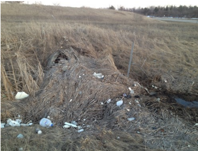
Figure 2-18: Blocked inlet
