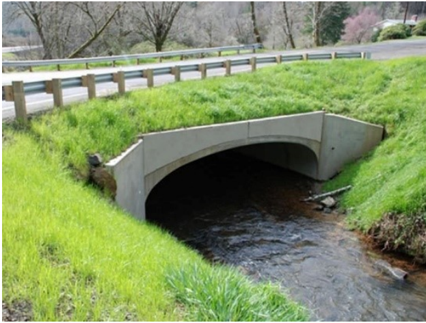
Figure 2-25: Concrete headwall and metal sheet pile wingwalls
