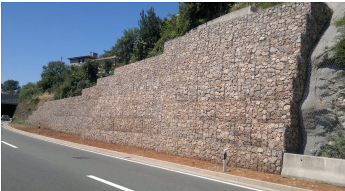
Figure 3-34: Gabion wall
