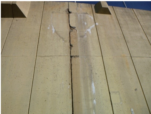
Figure 3-15: Efflorescence accumulation
