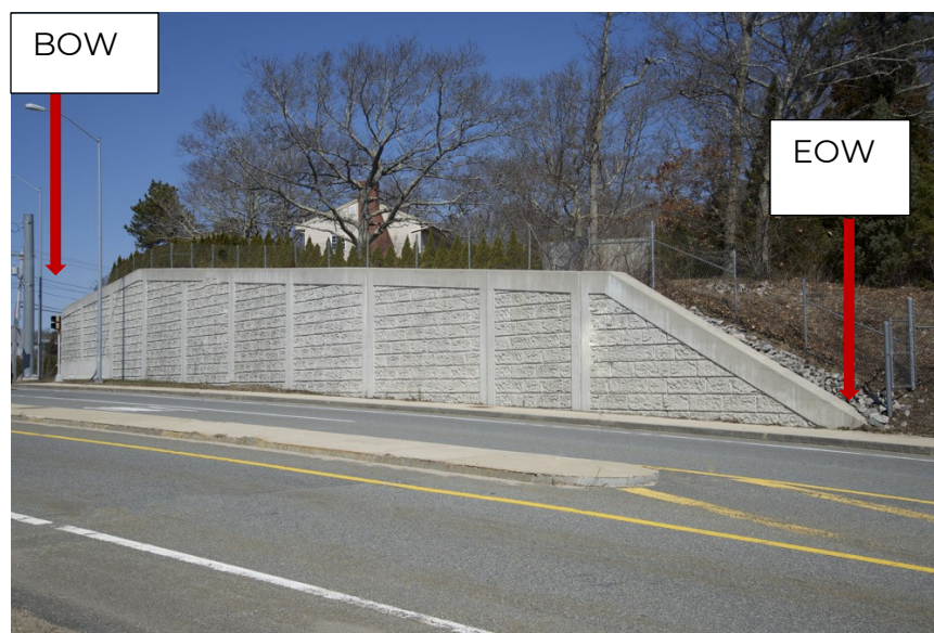
Figure 3-8: Typical wall facing inspection limits
