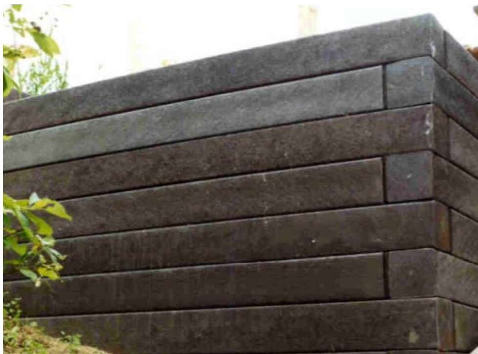
Figure 3-35: Plastic/vinyl lumber wall
