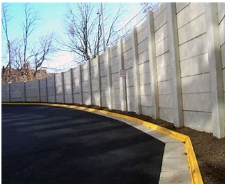
Figure 3-39: Vertical support concrete
