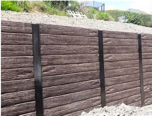
Figure 3-38: Vertical support steel
