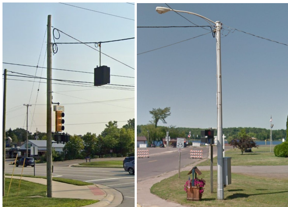
Figure 5-9: Embedded wood pole (left) and embedded steel pole (right)
