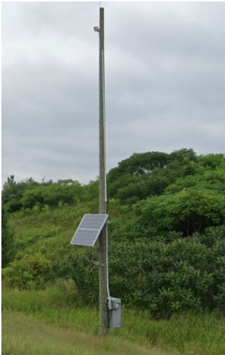
Figure 5-3: Embedded wood pole supporting ITS infrastructure
