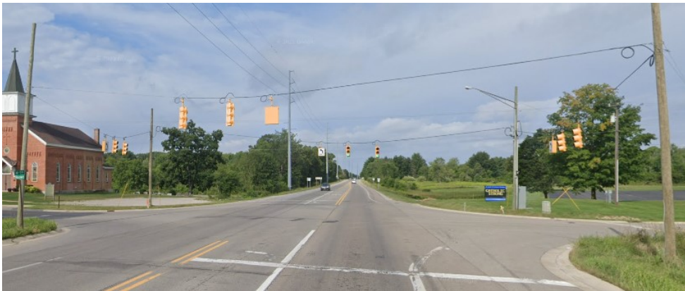
Figure 5-1: Embedded wood poles with box span configuration
