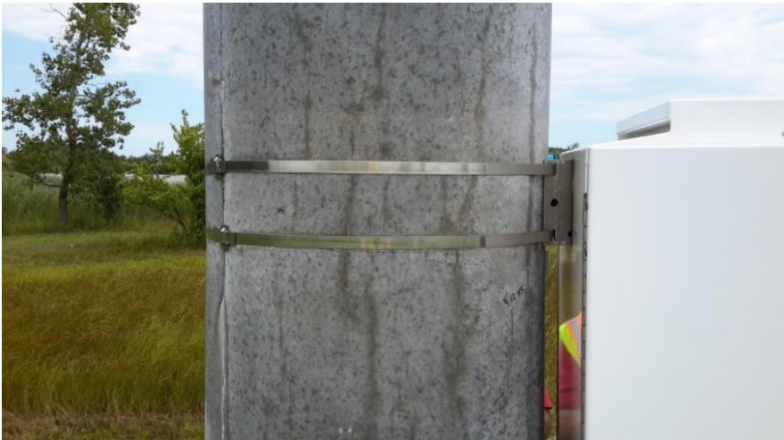
Figure 6-7: Band clamp connection to metal enclosure
