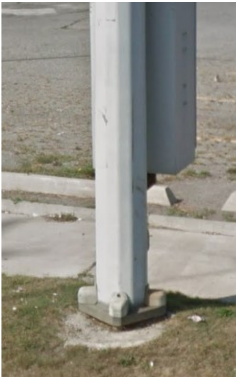
Figure 7-6: Steel strain pole (multi-sided) structure with four anchor bolts (left) and six anchor bolts (right)
