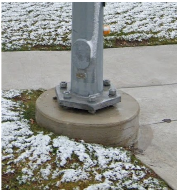
Figure 7-6: Steel strain pole (multi-sided) structure with four anchor bolts (left) and six anchor bolts (right)
