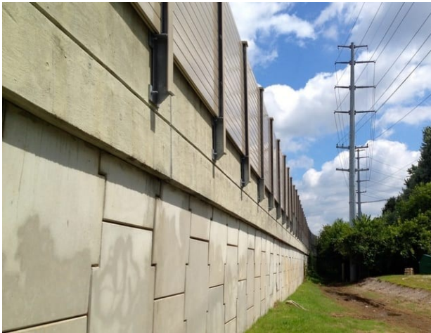
Figure 8-11: Noise wall attached to retaining wall
