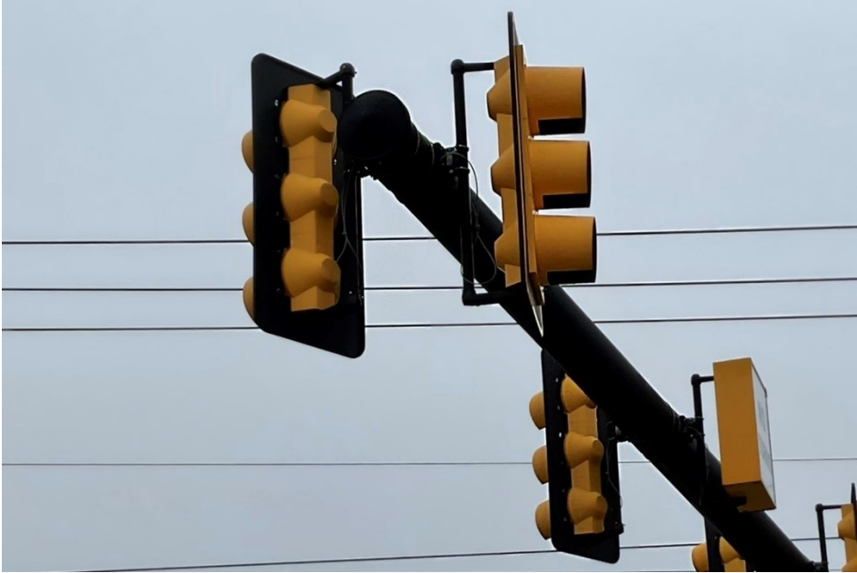
Figure 9-16: Mast arm signal and sign attachment connections
