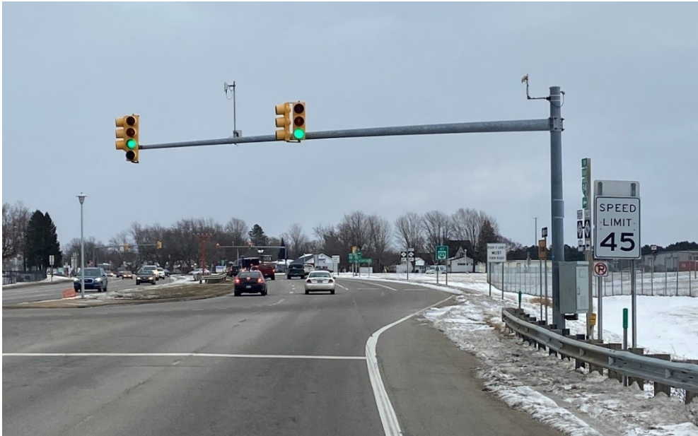
Figure 9-14: Mast arm structure with single arm
