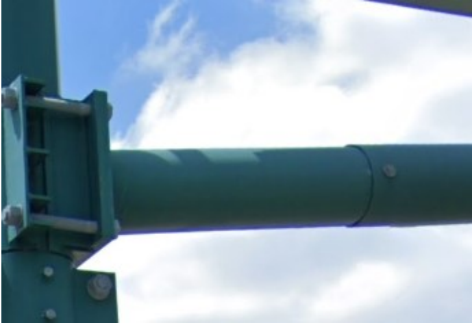
Figure 9-15: Mast arm member splice with connection bolt
