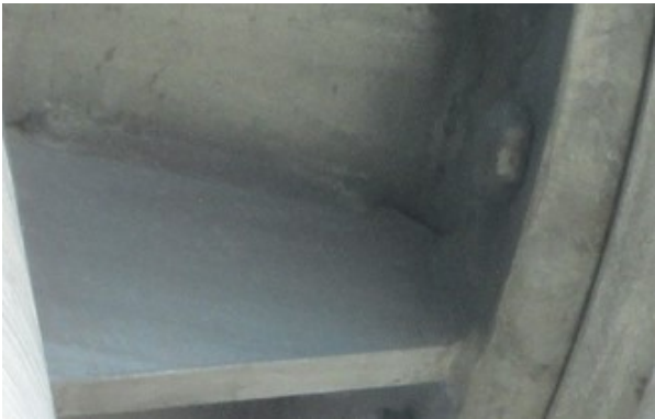
Figure 10-12: Vertical structure connection, missing flat washer on head side of bolt
