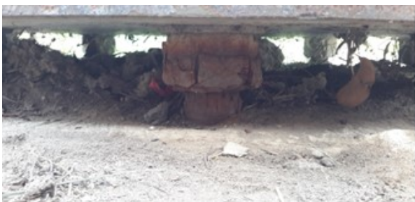
Figure 10-8: Leveling nut and anchor bolt corrosion with section loss
