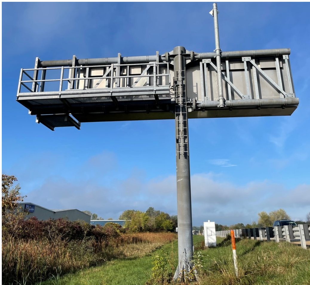
Figure 10-3: Dynamic Message Sign Support Structure
