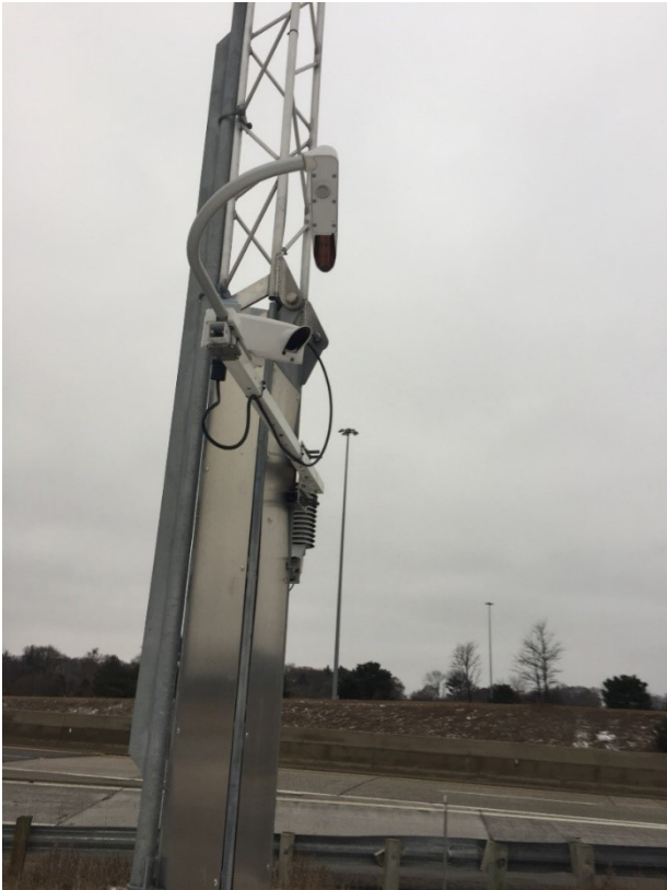
Figure 14-7: ESS tower vertical support column with ITS attachments
