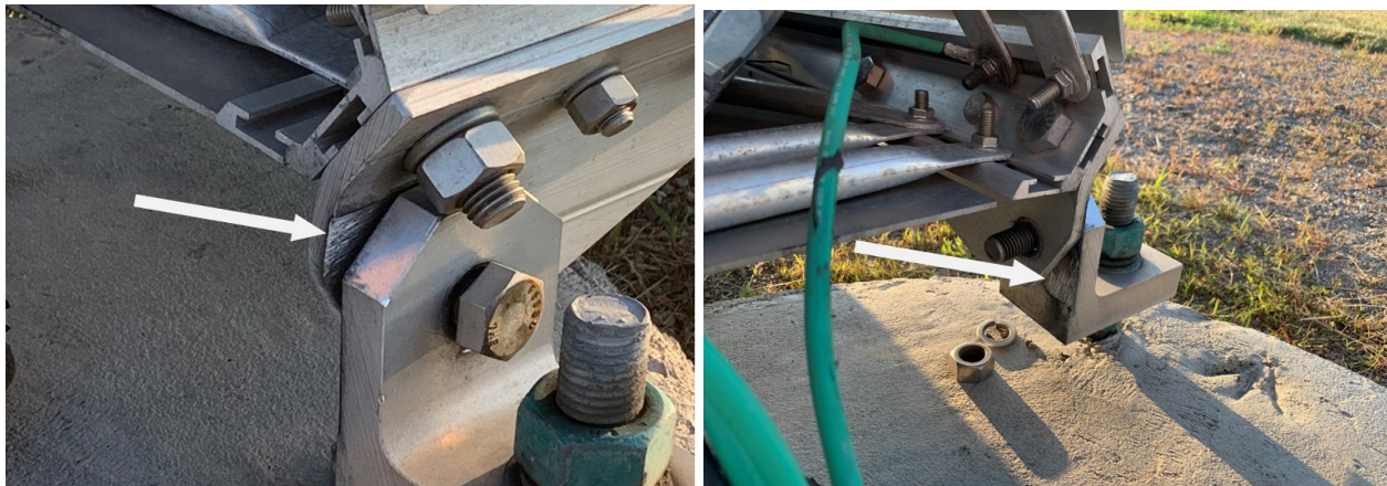
Figure 14-9: Evidence of wear on metal due to oscillation along with loose connection
