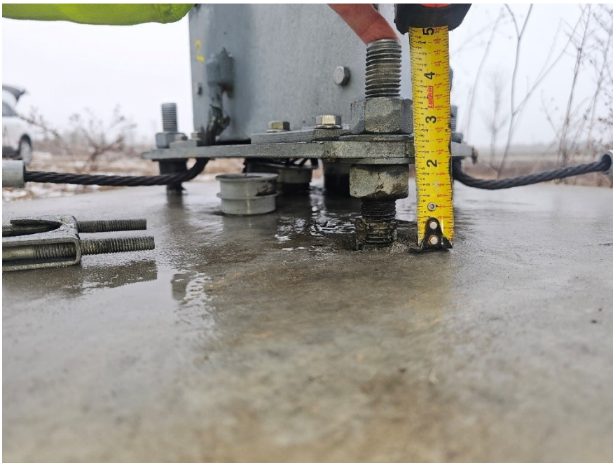
Figure 14-5: Standoff measurement for a sound foundation
