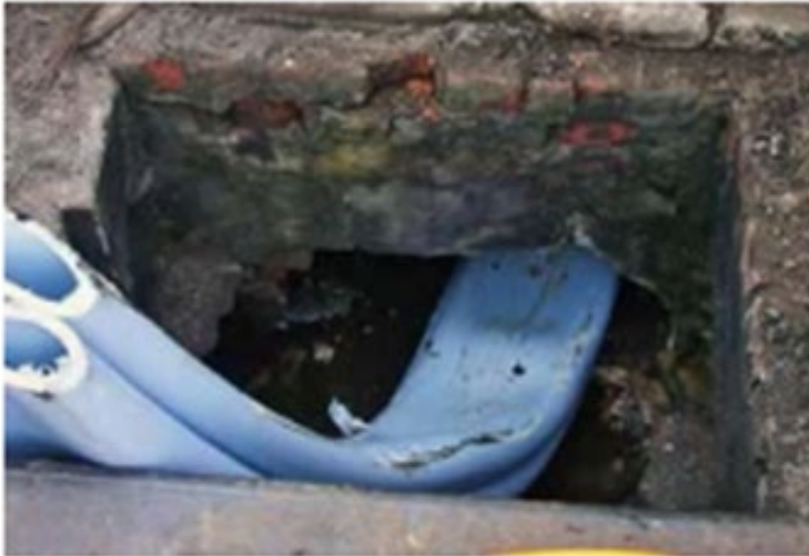
Figure 12: Fold-and-Form Liner: Liner Protruding (left) and Steam Pressure to Re-round PVC Liner (right)
