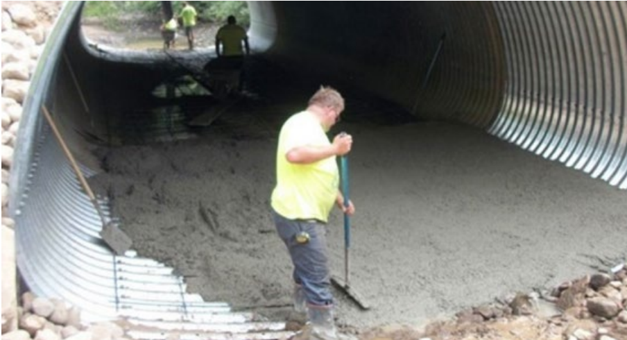
Figure 22: Invert Paving of a Corrugated Metal Arch Pipe
