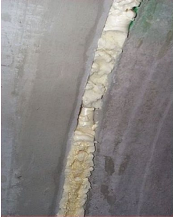
Figure 1: Internal Side of a Chemically Grouted RCP
