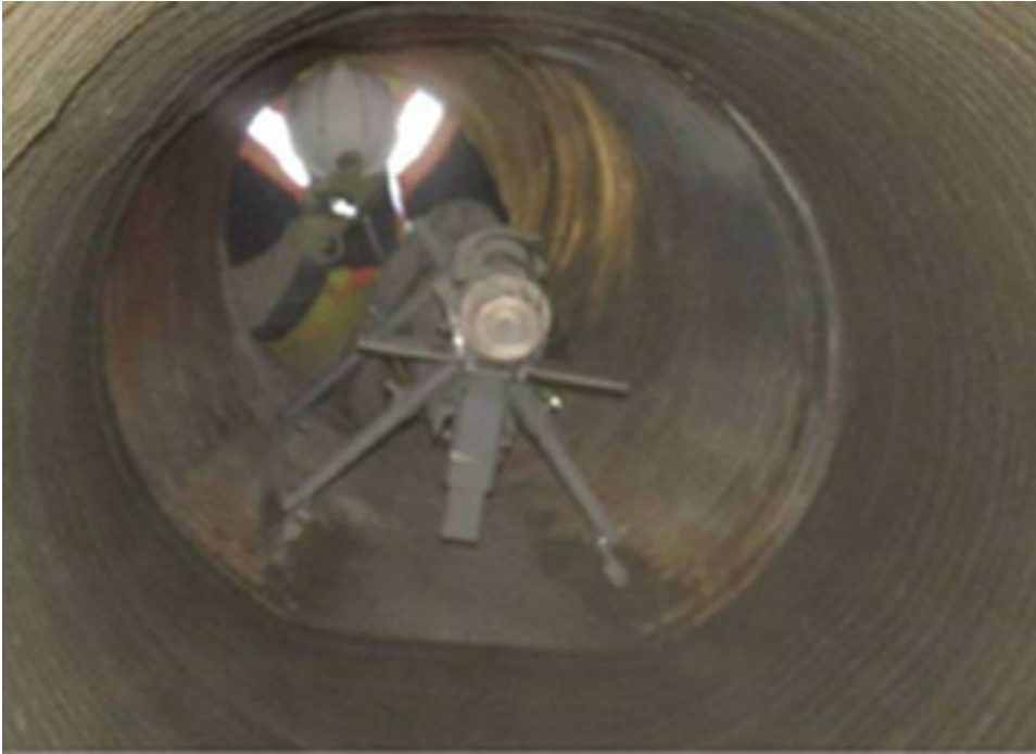
Figure 18: Installation of Centrifugally Cast Liner
