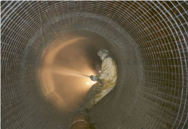
Figure 4: Internal Shotcreting through Human Entry
