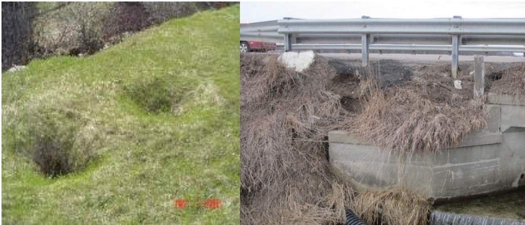
Figure 2-11: Example of embankment issues due to piping (left) or erosion (right)
