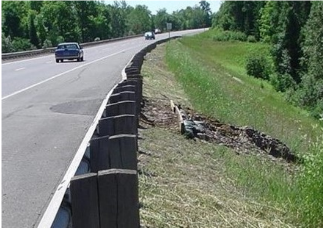
Figure 2-11: Example of embankment issues due to piping (left) or erosion (right)
