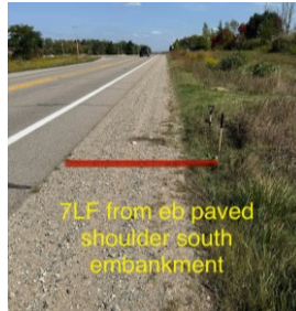
Sinkhole over open culvert joints
