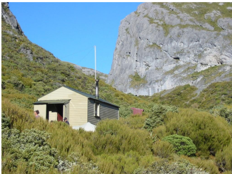
Left: Granity Pass Hut, Ghost Valley, North Owen
