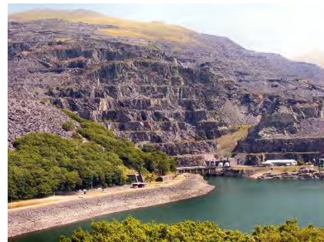
Figure B2-1: Dinorwig Power Station
