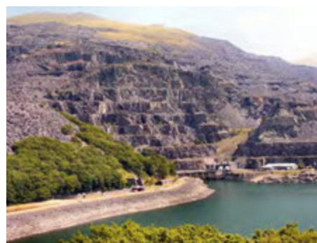
Figure B2-1: Dinorwig Power Station
