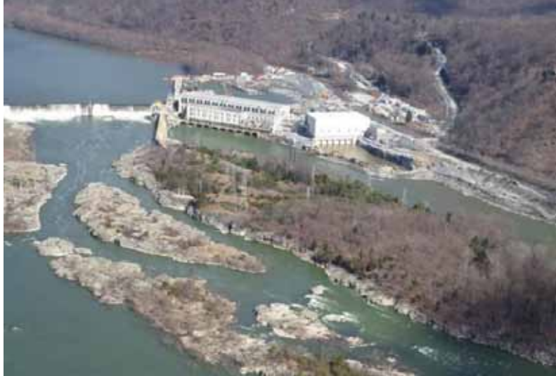
New turbines were installed at Holtwood hydropower station last year, bringing its capacity from 107MW to 232MW
