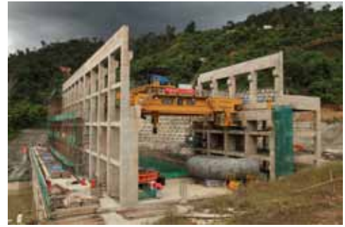
Murum Construction Site (Power House)
