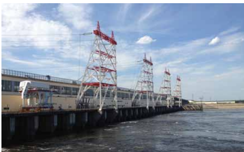
Cheboksarskaya Hydropower Plant, Russia (Photo: IHA)
