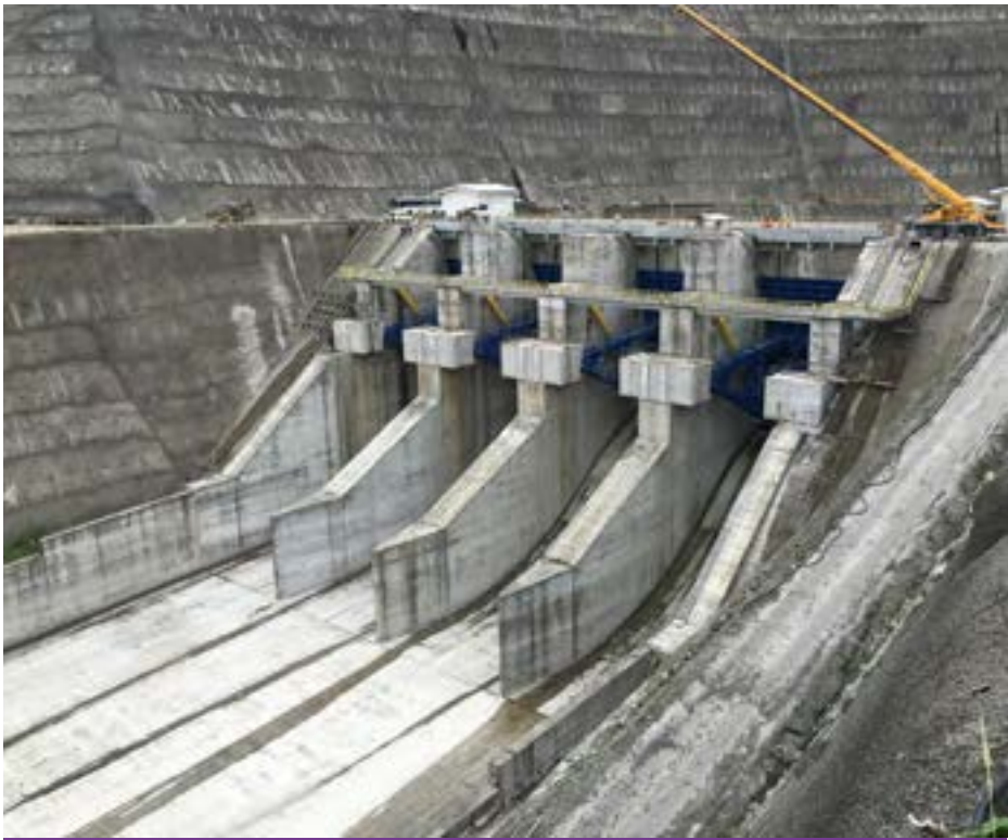
Construction of the dam at Reventazón
