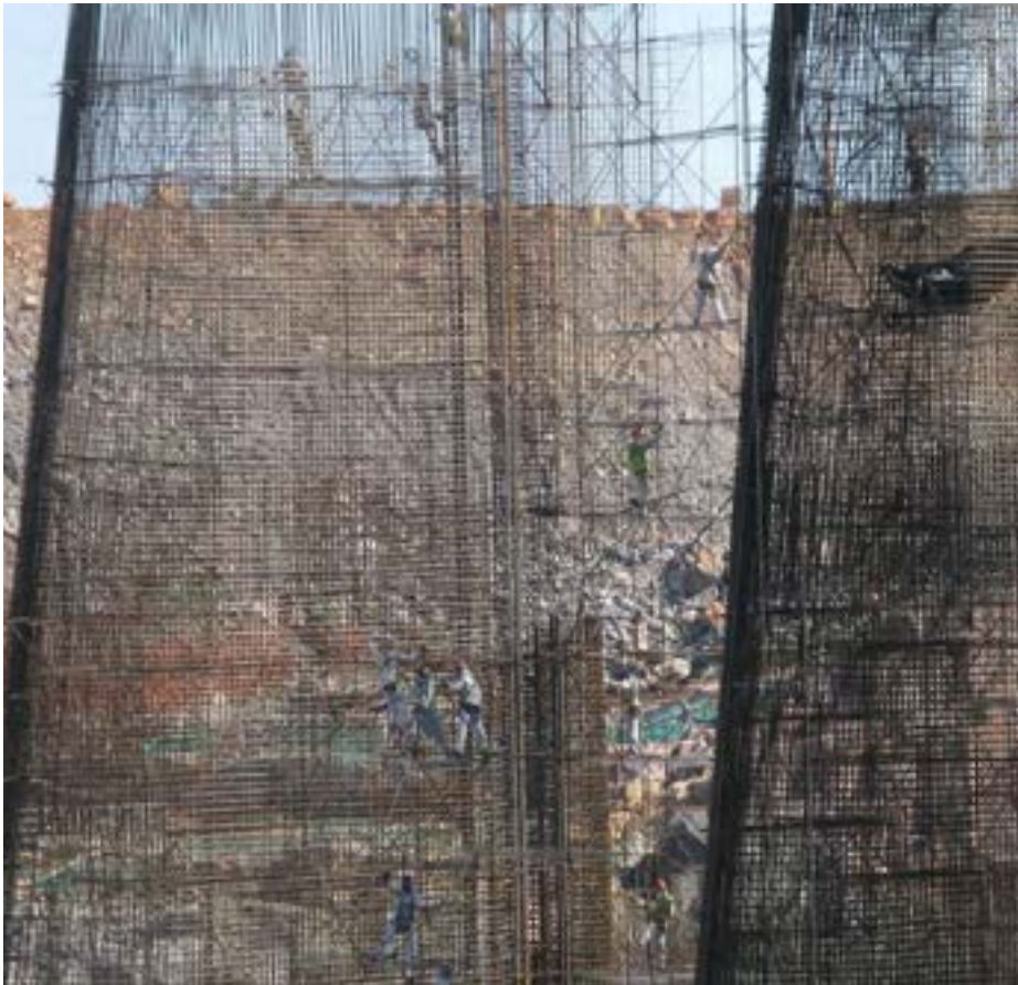
Construction workers at the Santo Antônio project
