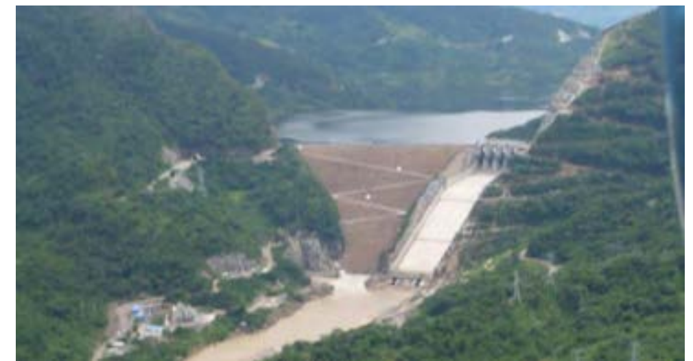
The site of the Sogamoso hydropower plant
