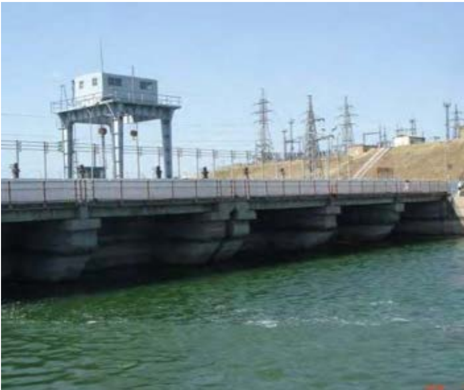
Shardara hydropower plant
