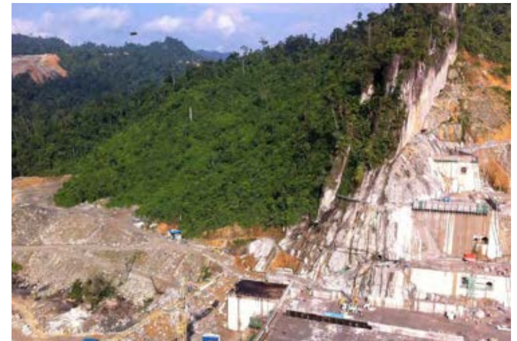
Construction of the Murum project
