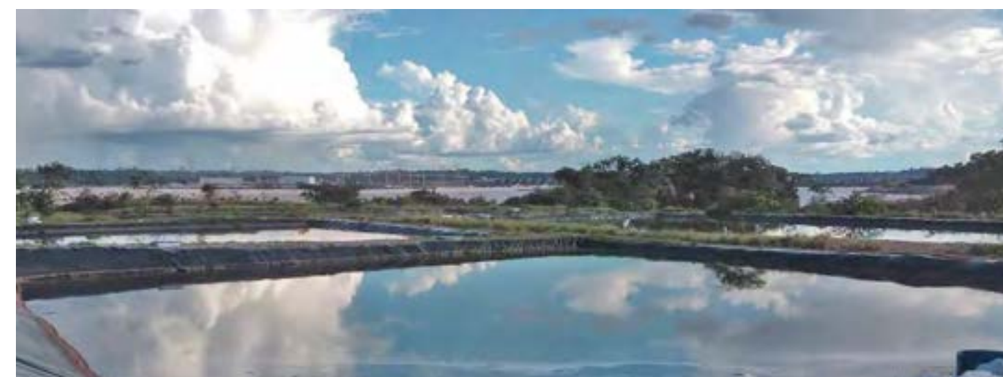
Water treatment ponds
