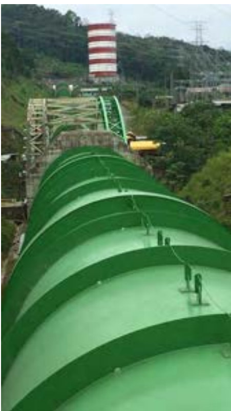
The powerhouse penstock and surge tower
