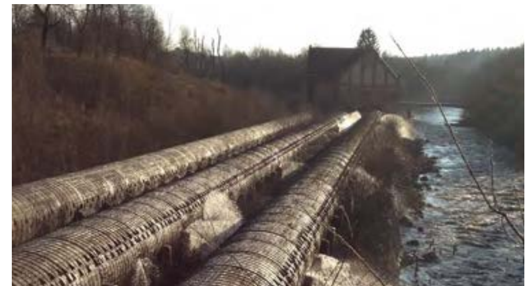
Penstocks of the existing Semla plant, which are leaking badly and will be replaced by one new penstock with the construction of Semla IV
