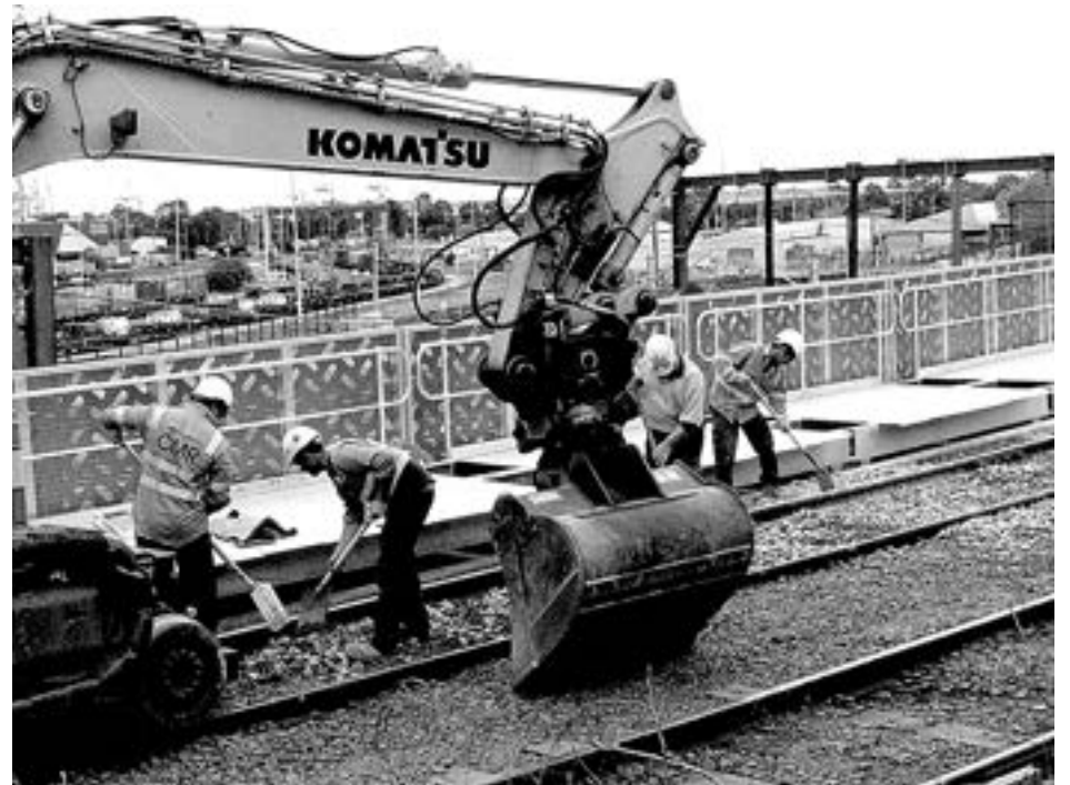
Regional Rail workers construct emergency footpaths and install handrails on the flyover
