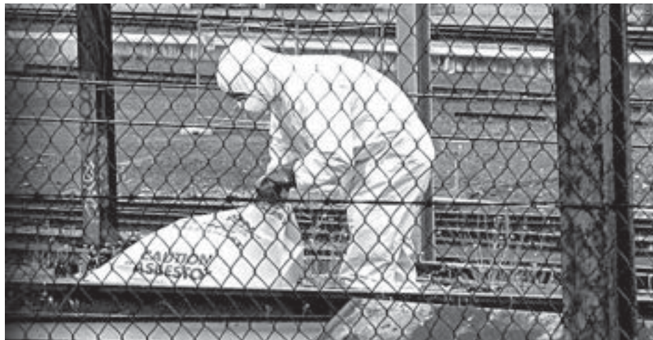
A Regional Rail Link employee removing asbestos from Railway Place tracks on Good Friday
