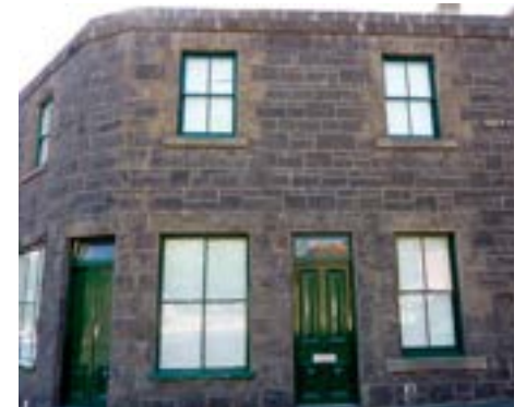
A solid bluestone masonry building on the corner of Chetwynd and Stanley streets. The location, the multiple windows and sturdy construction suggest this is a pub or inn, dating back to 1870 or earlier. This is mainly a workers' establishment, and possibly a bit rough for the middle class patrons down the road. Masonry of this quality and volume was only used when it was absolutely necessary, due to the laboriousness of stone cutting and laying. It acts as fire protection as well as protection from violent intruders.
