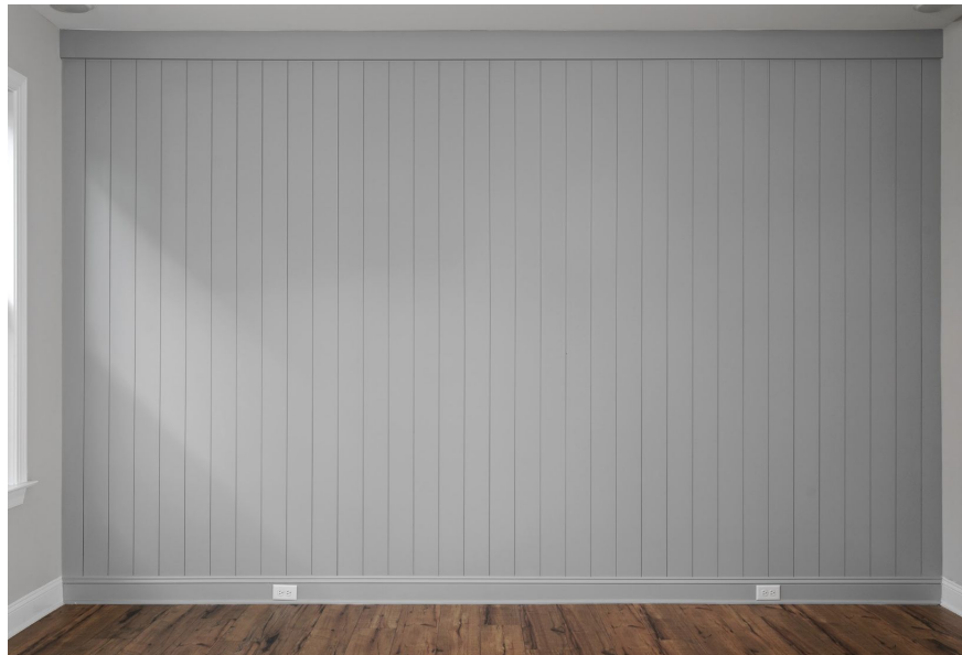
EXAMPLE: VERTICAL SHIPLAP WALL PRIMARY BEDROOM
