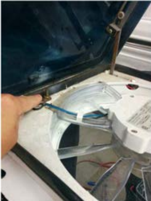
Exterior vent switch PHOTO F-6
