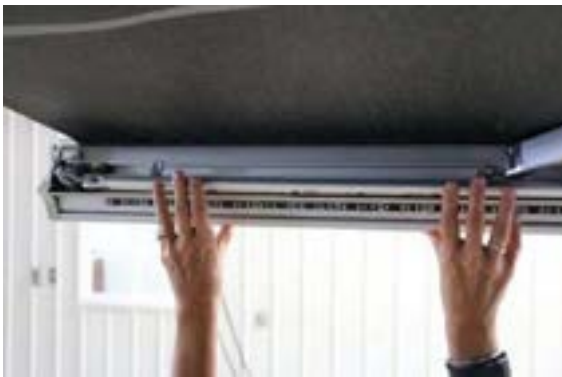
Vertical supports PHOTO F-15
