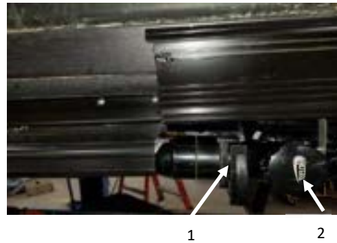
Wastewater drainage PHOTO D-35
