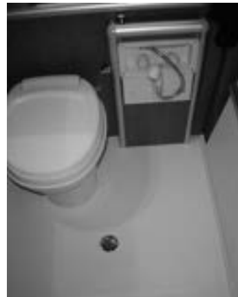
Floor raised PHOTO D-21
