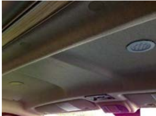
Reading lights PHOTO E-1
