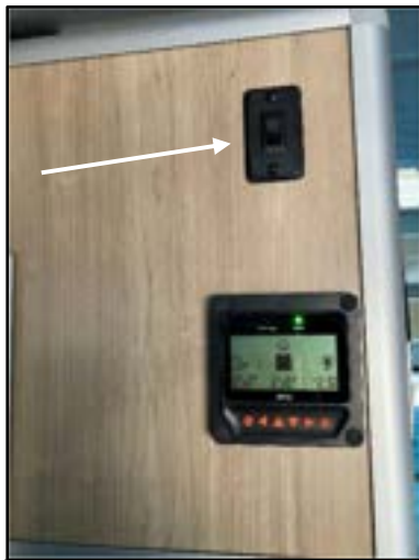
PHOTO K-5 Electric bed switch
