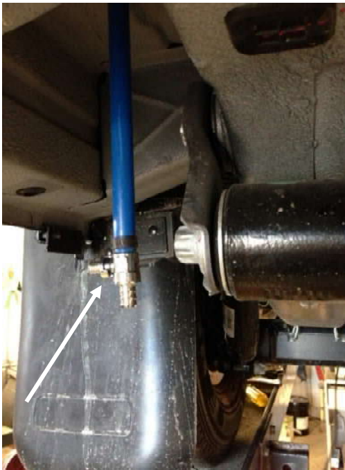
Potable water tank valve PHOTO D-7
