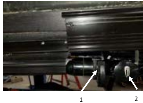
Wastewater drainage PHOTO D-35
