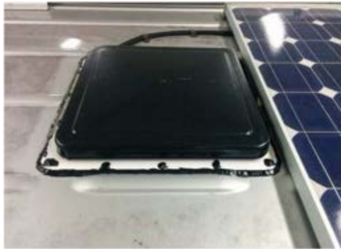
Vent gasket PHOTO F-7
