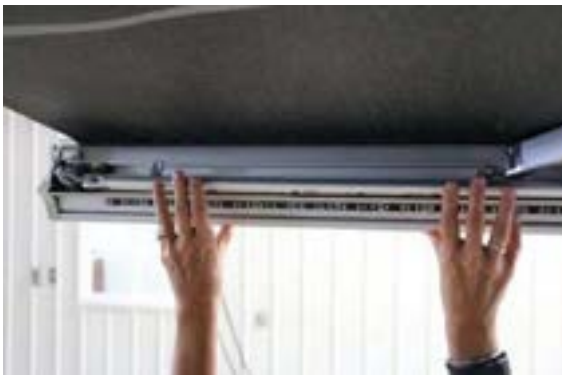
Vertical supports PHOTO F-15
