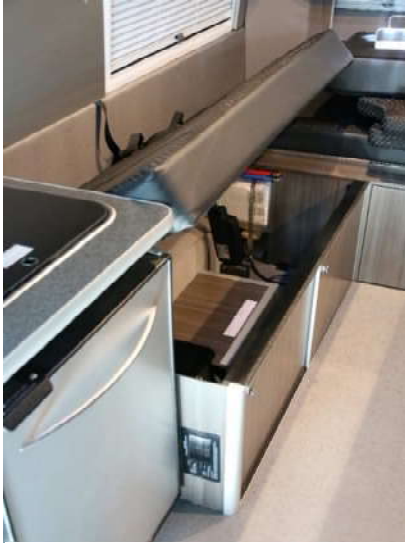
Motor under bench PHOTO E-47
