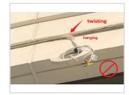
Do not allow light fixture to hang or twist while installing into mounting profile. Improper handling could lead to damage to the internal PCB of the fixture.
