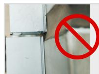
Do not join mounting profile in the same location as the wall joints. The expansion and contraction of the building surface will pull the lighting connection apart. Damage to components can result.
