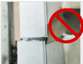
Do not join mounting profile in the same location as the wall joints. The expansion and contraction of the building surface will pull the lighting connection apart. Damage to components can result.
