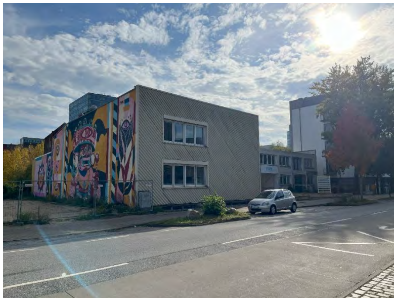
Figure 2A view from the backside of the building
