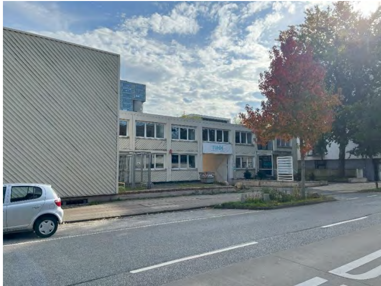
Figure 1A view from the entrance and external view of the building
