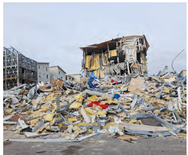
Earthquake damage in the hardest-hit state of La Guaira, where 80% of structures collapsed.
