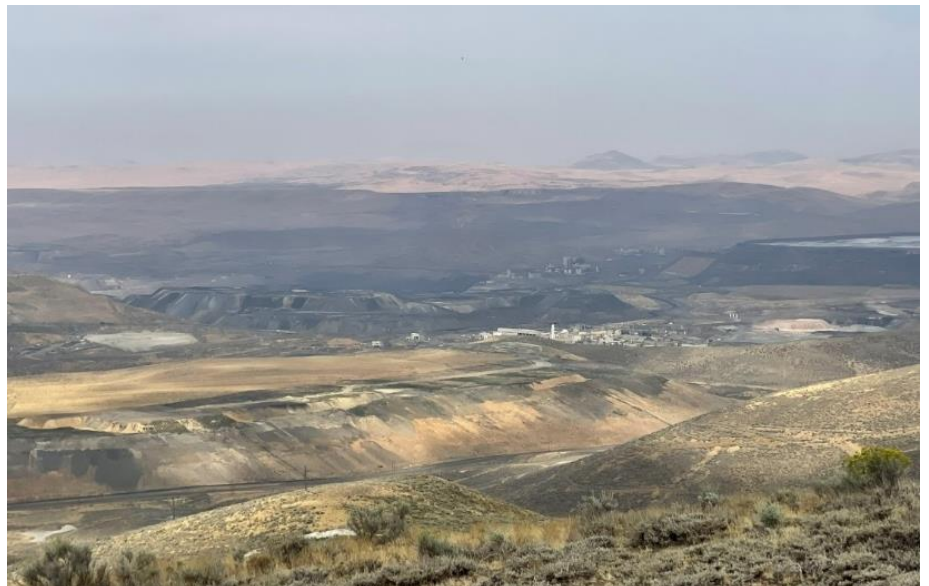
Figure 70: Carlin heap leach pads (foreground), roaster/autoclave (middle ground) and tailings dam (background)
