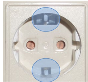
[Electrical outlet grounding position]
