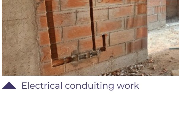
Electrical conduiting work
