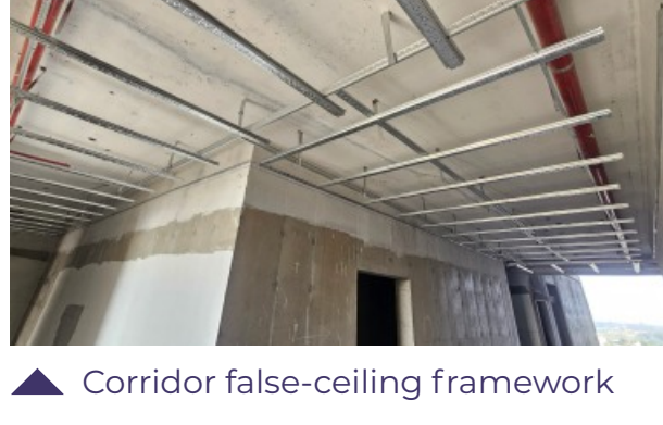
Corridor false-ceiling framework
