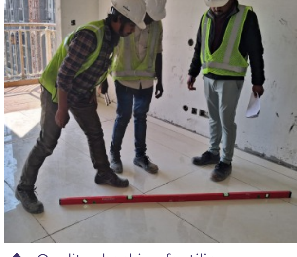
Quality checking for tiling
