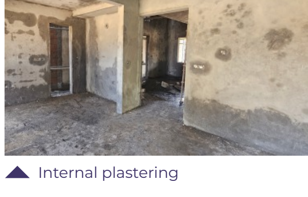
Internal plastering
