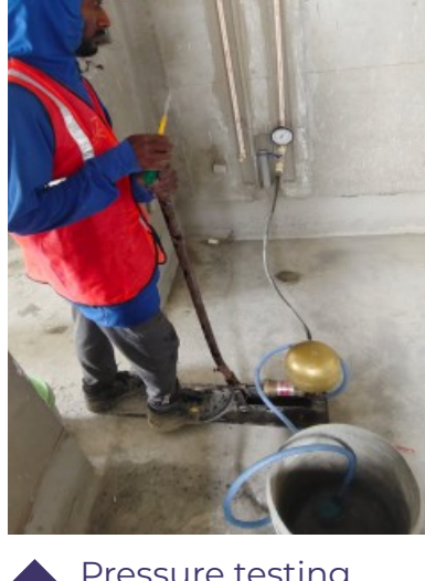
Pressure testing for pipelines
