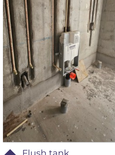
Flush tank installation
