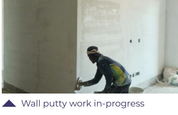
Wall putty work in progress
